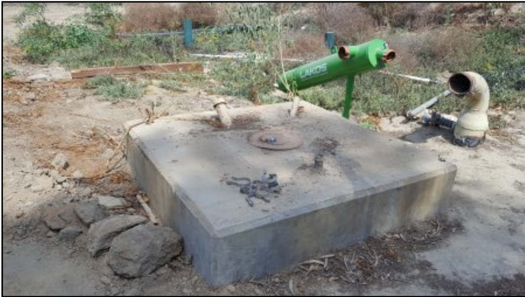
8 : View of capped well and sand filter north of pond.
