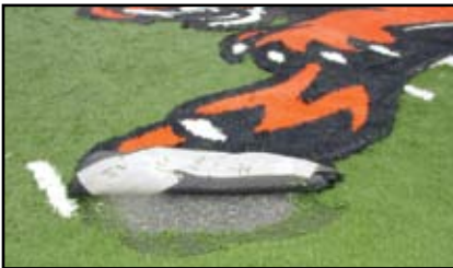
Installation of a special logo on a synthetic field. Photo: Darian Daily
