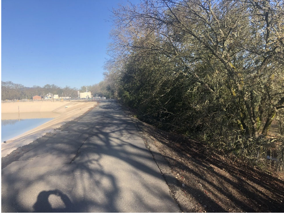
Photograph 1 View northwest of developed areas and oak woodland from the eastern portion of the study area.
