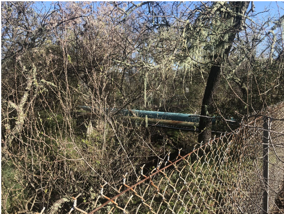
Photograph 4 View southwest of existing pipeline crossing over Simmons Creek and surrounding riparian woodland.
