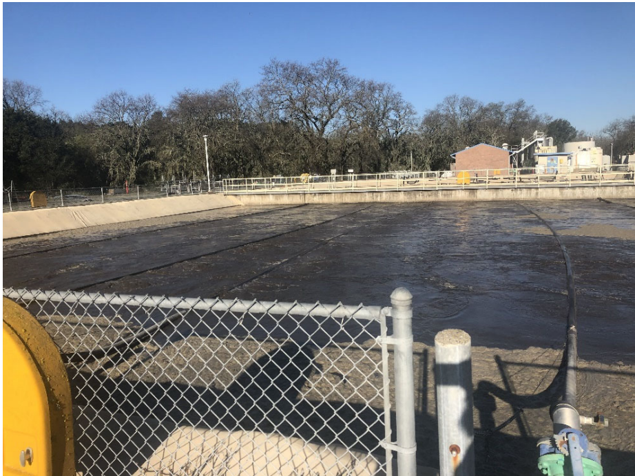
Photograph 2 View west of the developed areas within the eastern portion of the study area.
