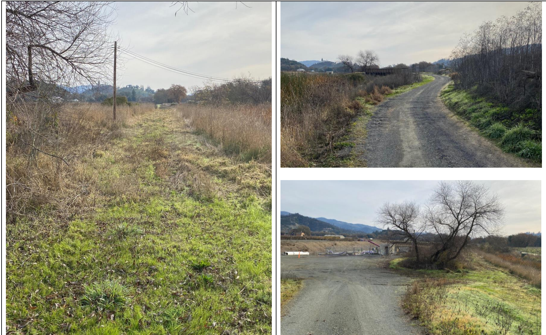
Figure 2 Existing Temporary Access Road Conditions (December 2023)
