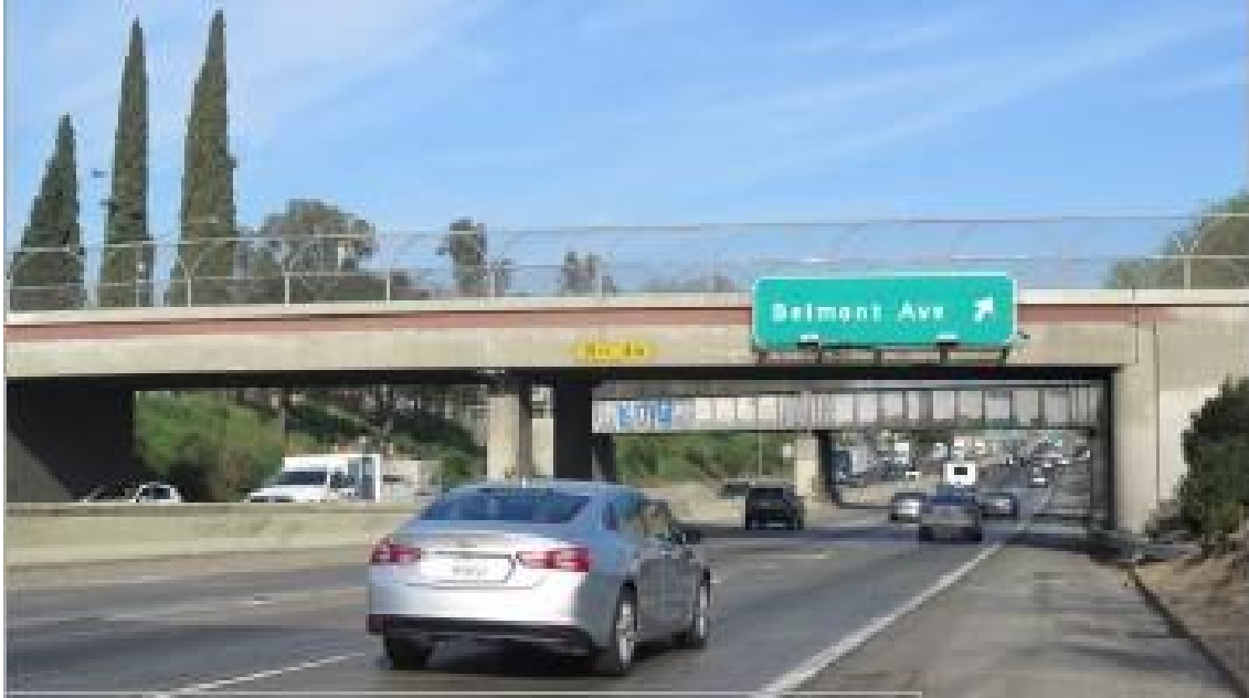
Figure 2-17 Existing Teilman Avenue Overcrossing and Kerman Avenue Underpass
