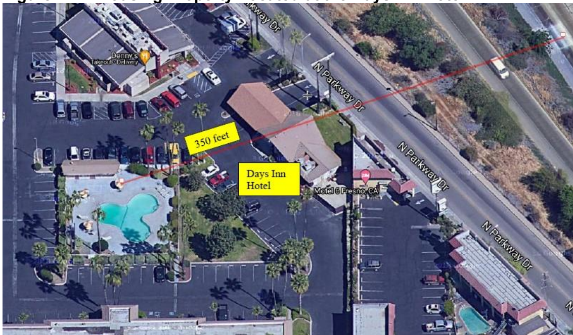
Figure 2-27 Housing Property Located at the Days Inn Hotel
