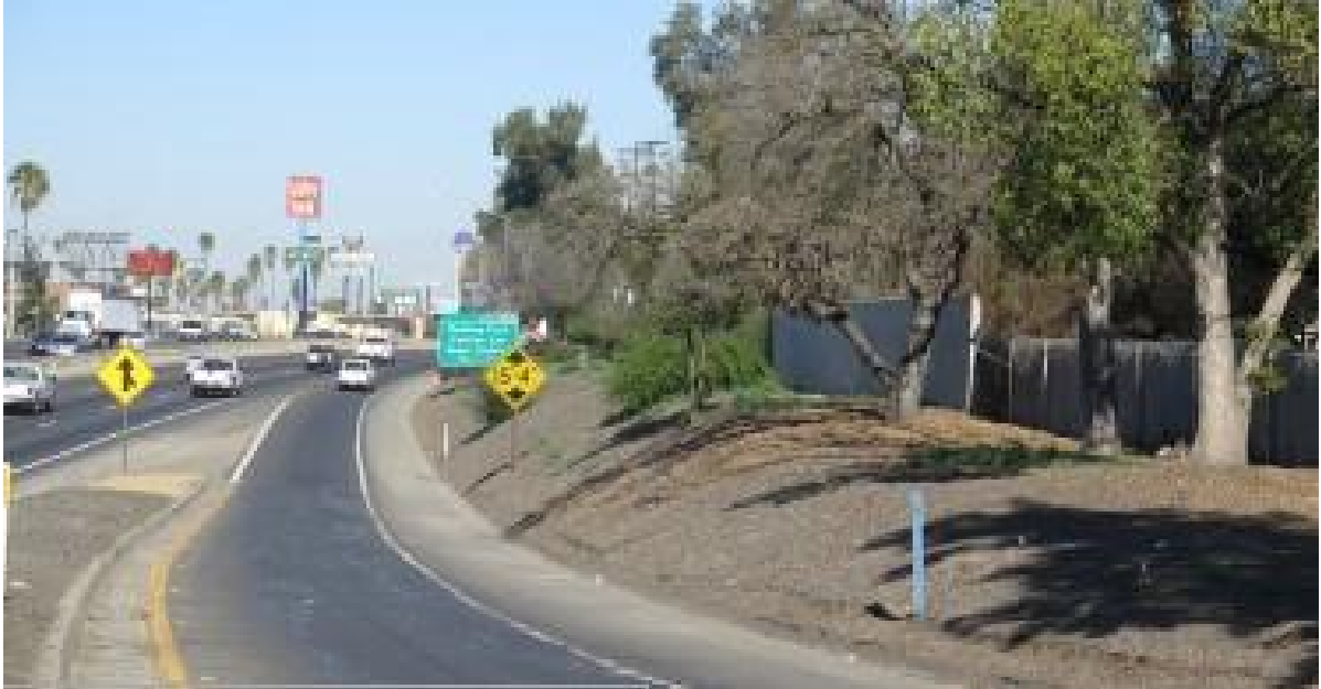
Figure 2-18 Existing Condition of State Route 99 at Belmont Avenue, Facing North at Roeding Park
