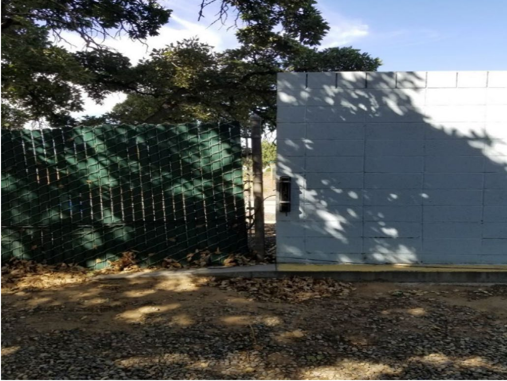
Figure 2-30 South End of Existing Soundwall/North End of Chain Link Fence
