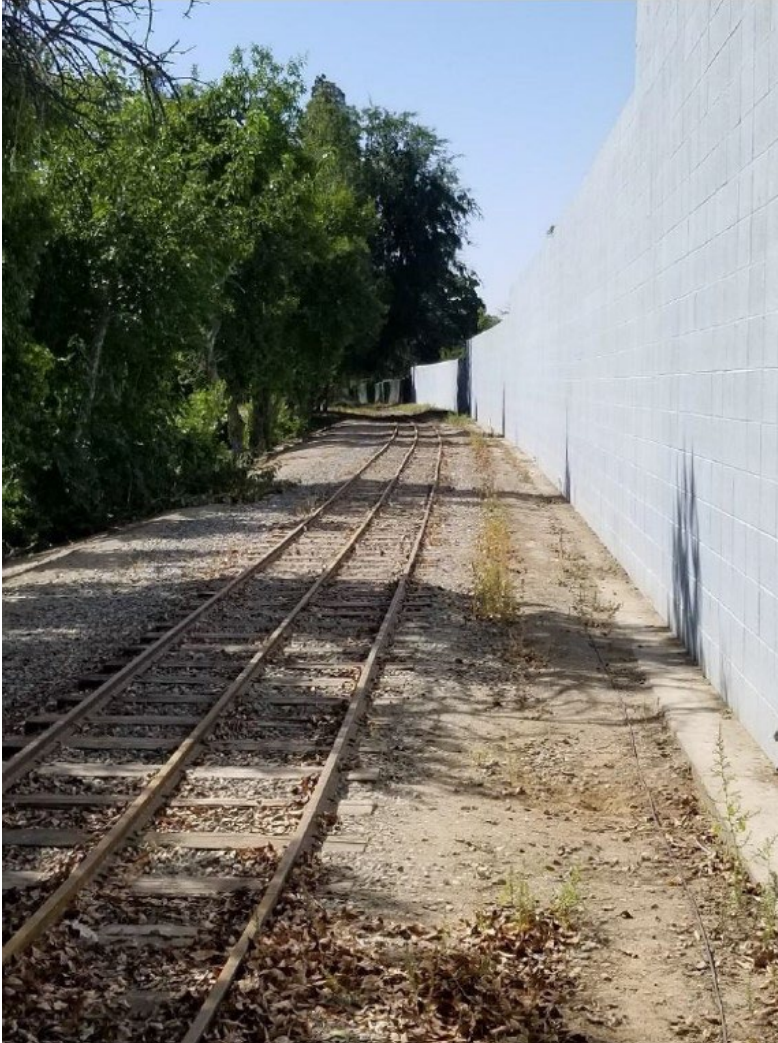
Figure 2-34 Existing Soundwall Within Roeding Park
