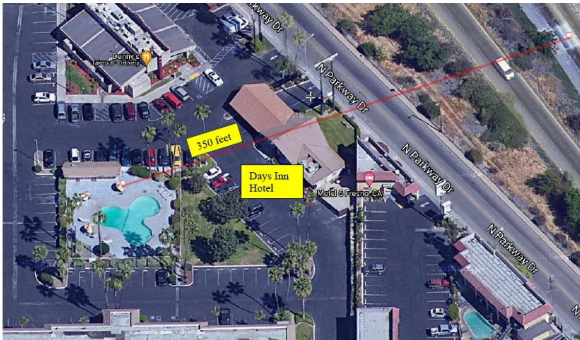
Figure 2-27 Housing Property at the Days Inn Hotel
