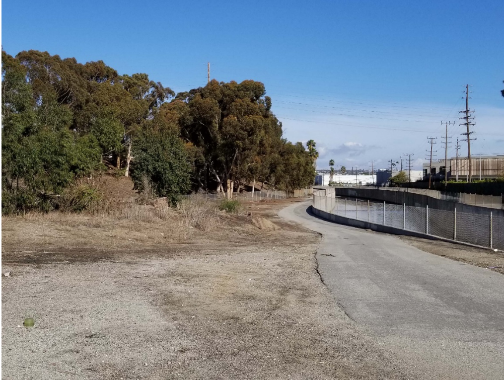
Figure 2. Access road, view toward northeast.
