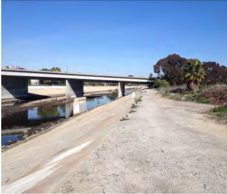
Photograph 3 Facing North East
