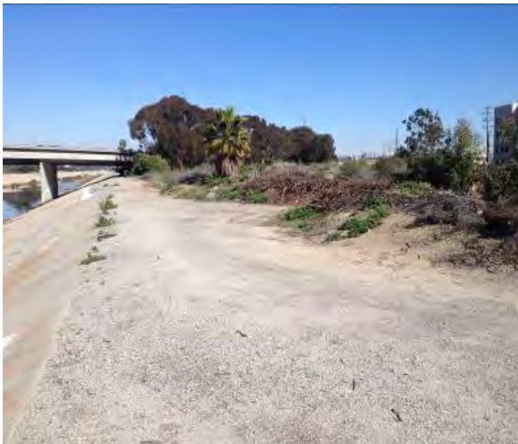
Photograph 4 Facing North East.
