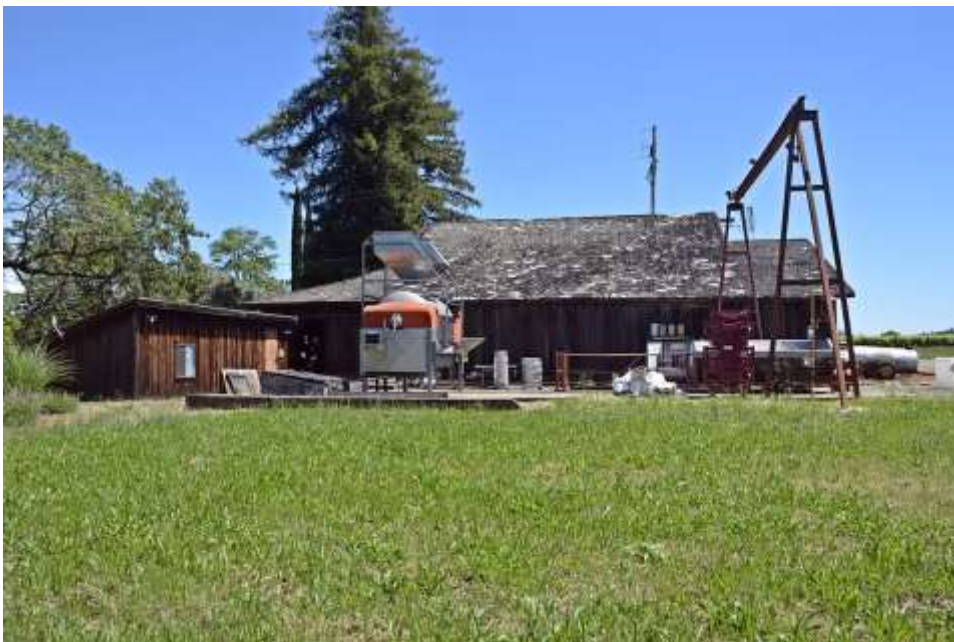
Photo 17: North elevation with non-historic crush equipment in foreground. Camera facing southeast.
