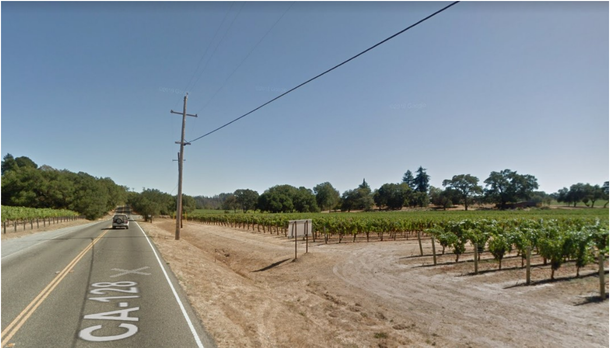
VIEW OF PROJECT SITE IN DISTANCE FROM THE SOUTH ON HIGHWAY 128
