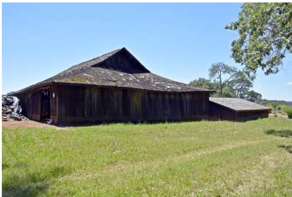
Photo 15: East elevation showing hipped roof section. Camera facing southwest.
