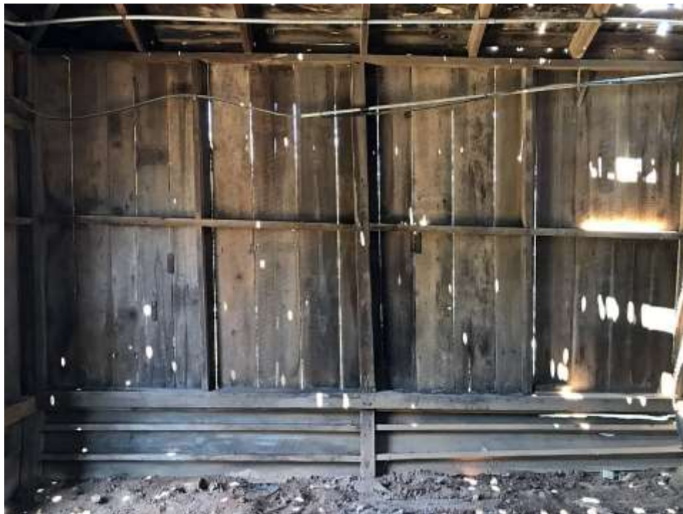
Photo 18: East wall showing light wood-frame construction and raised section below.
