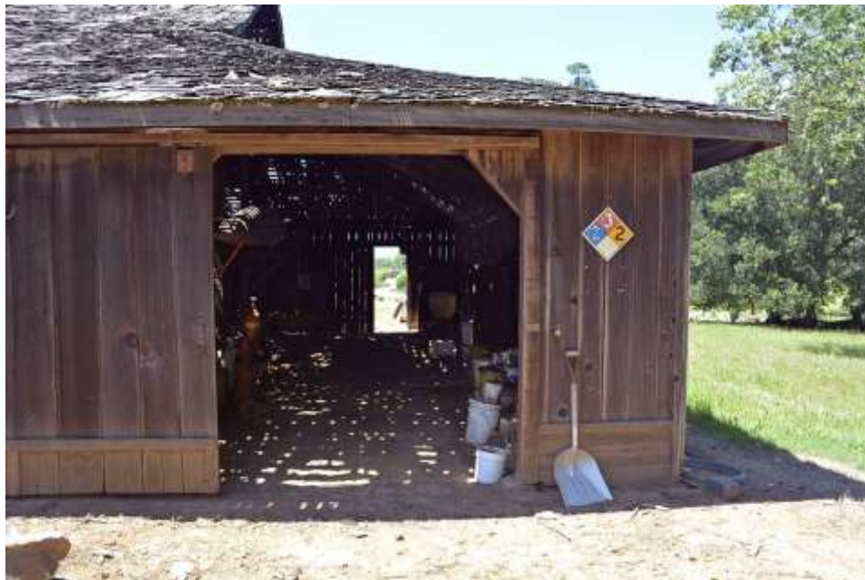
Photo 14: South elevation showing drive-through opening. Camera facing northwest.
