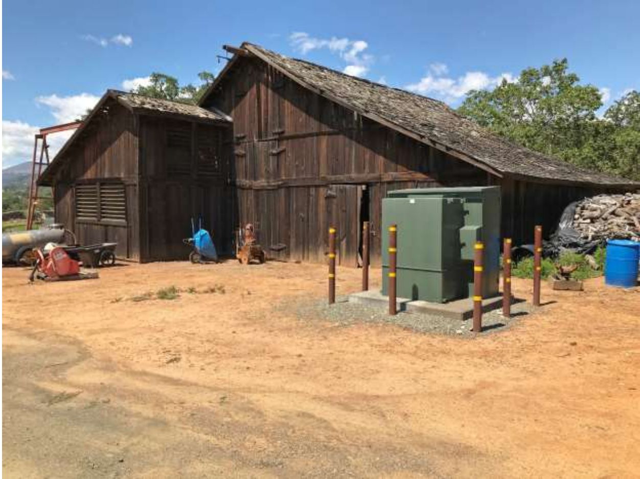
Photo 1: Subject Structure, Barn, aka, Field Stone Winery and Vineyard Barn. West, front elevation, facing northwest. John W. Murphey, May 28, 2019.
