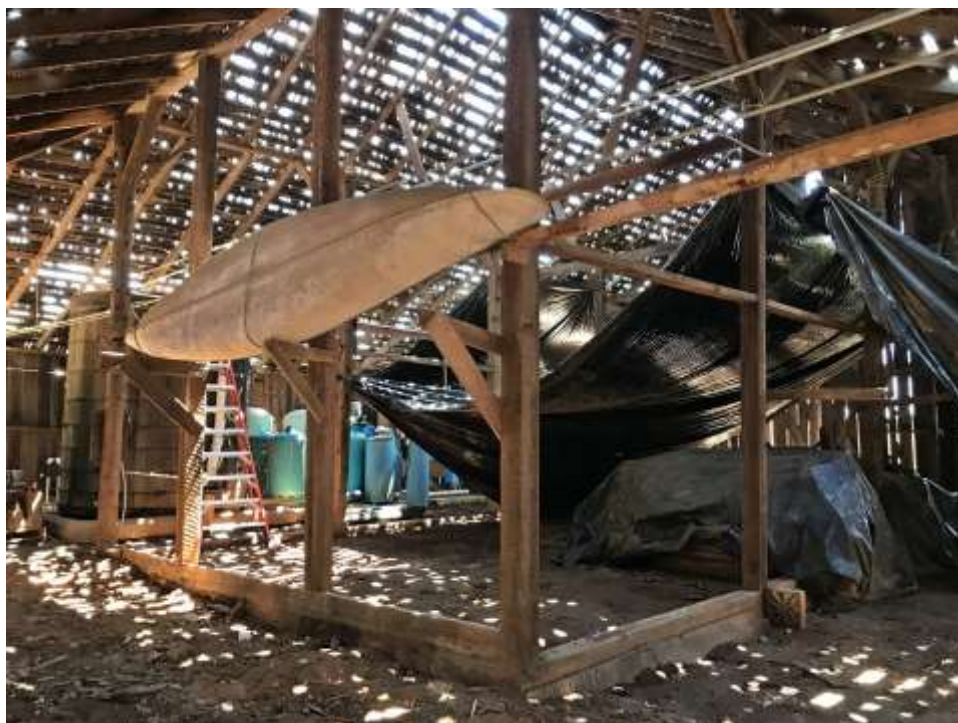
Photo 19: Three-bay core structure.
