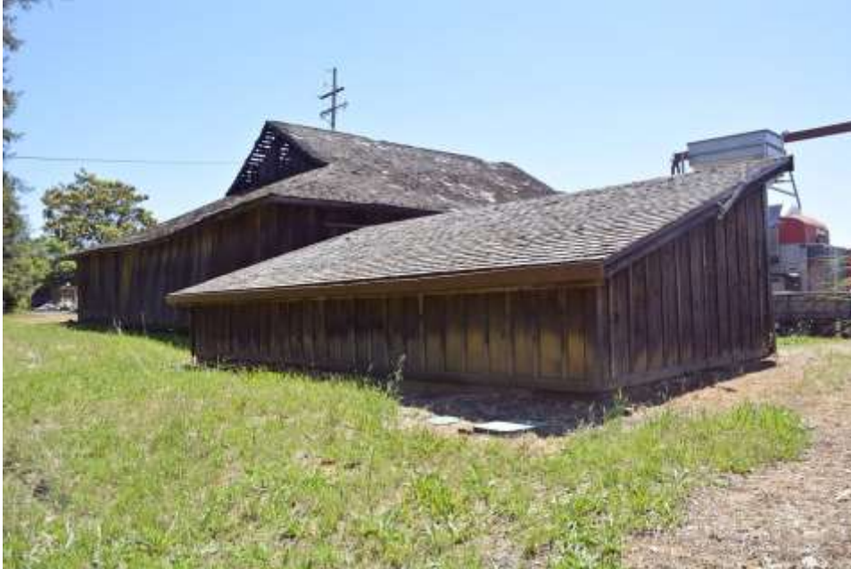
Photo 16: East elevation with non-historic shed in foreground. Camera facing southeast.
