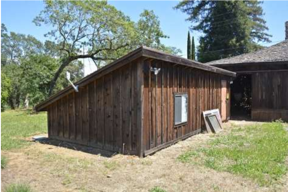
Photo 4: Non-historic shed. Camera facing northeast.
