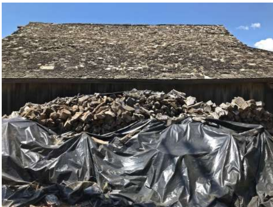
Photo 13: South elevation. Camera facing northwest.
