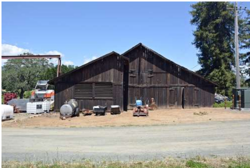
Photo 8: West (front) elevation. Probable non-historic addition at left. Camera facing north.
