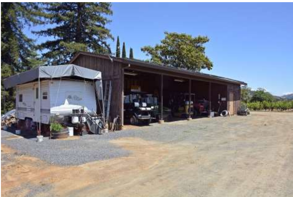
Photo 5: Non-historic equipment shed. Camera facing northeast.
