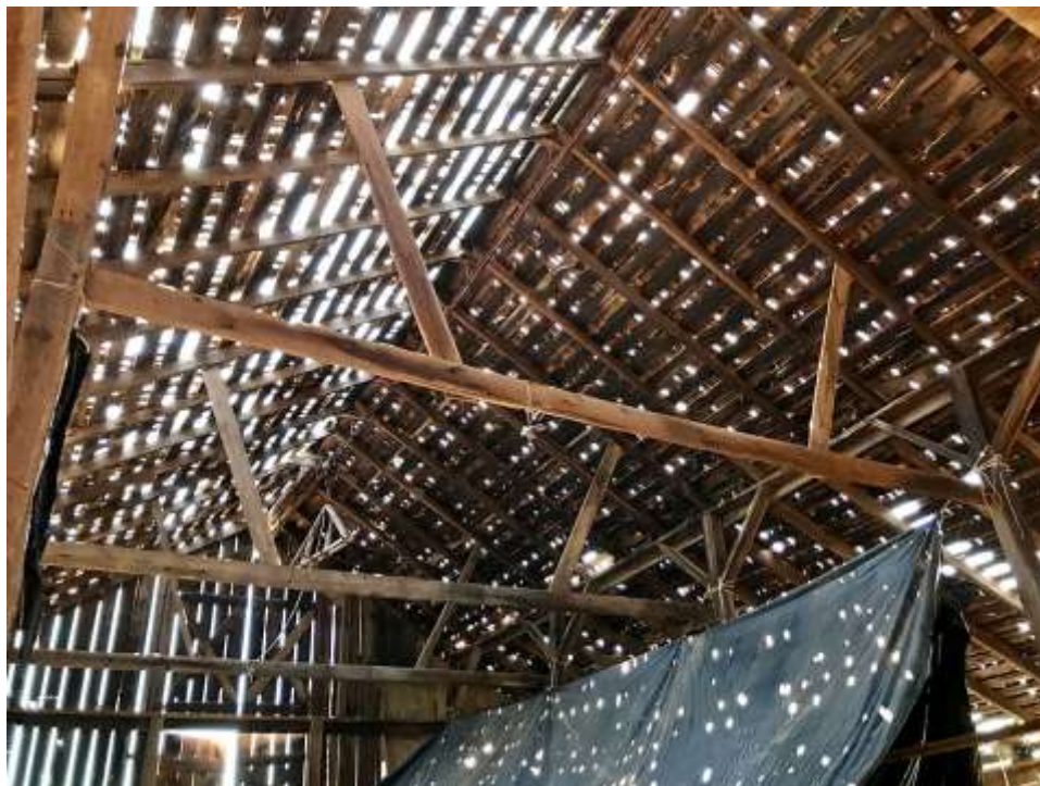
Photo 20: Trusses, rafters and roof boards.
