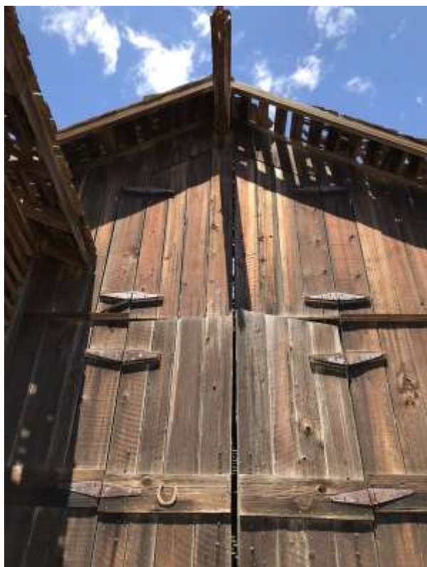
Photo 11: West elevation, hayloft doors. Camera facing up.
