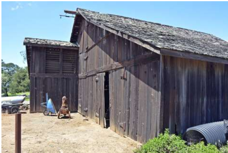
Photo 10: South elevation showing bump-out addition. Camera facing northwest.
