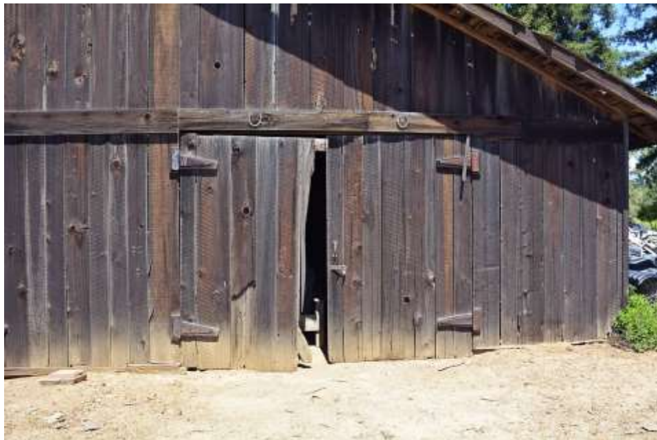
Photo 12: West elevation, vehicular doors. Camera facing northeast.
