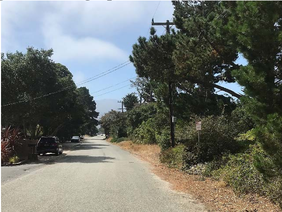
Photograph 1. Aerial Installation: Looking south from the northern end of Carmel Hills Drive.
