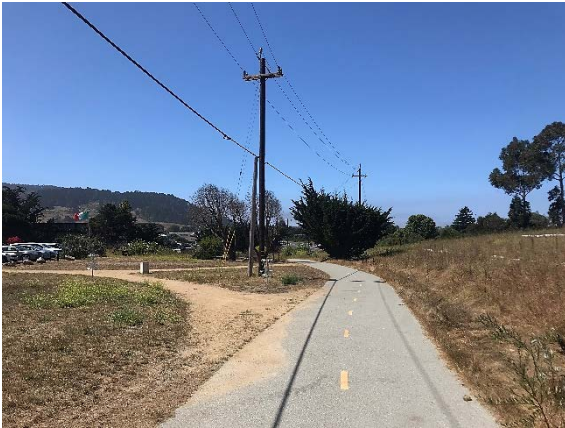
Photograph 3. Aerial Installation: Looking south along pedestrian/bike path near Barnyard Shopping Village.
