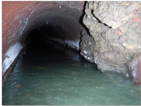
East Influent Pipe - 2336 Monroe St
