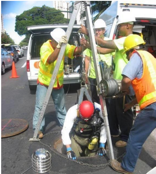
Photo 2-1. Confined Space Entry
