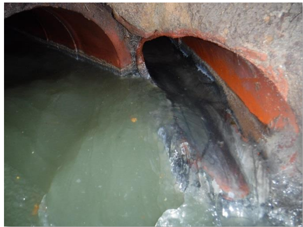
Southeast-East Influent Pipe and Southeast Monitored Influent Pipe - 2336 Monroe St
