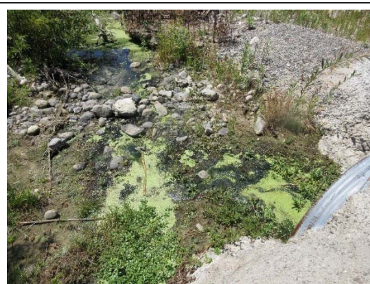
Discharge from the CAFO areas of the Riding Park could potentially contribute to existing water quality issues within San Juan Creek, which is considered an impaired waterway for indicator bacteria, phosphorus, total nitrogen, and other pollutants.
