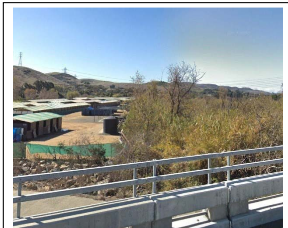
Development associated with the Riding Park, including the stables (left), is located in close proximity to San Juan Creek. Stormwater from the development has the potential to carry pollutants into the creek, which is currently listed under the CWA Section 303(d) List of Water Quality Limited Segments.
