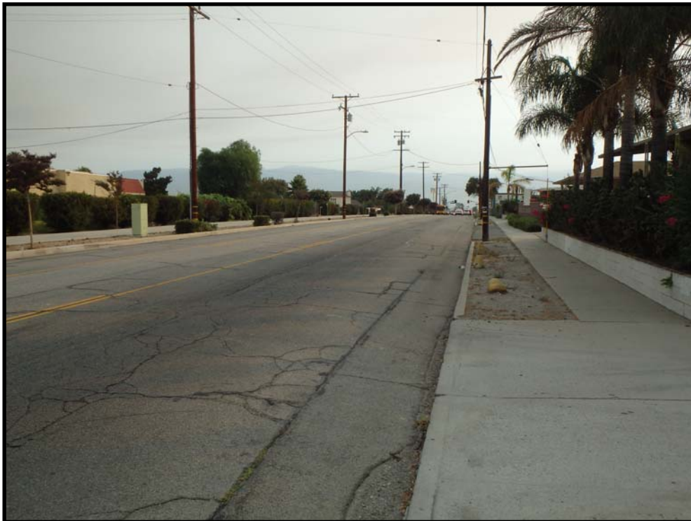
PHOTOGRAPH 2 - Inland Center Drive, where the stormdrain improvement will occur, looking northeast.
