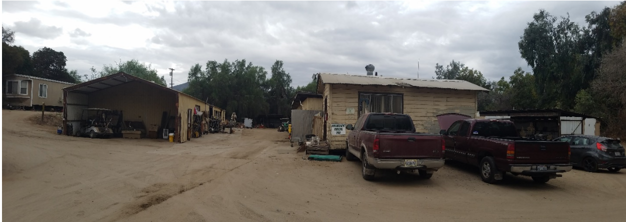
Figure 3. Maintenance facility, office shack in center, facing SW (EC-06, 11/19/2019)
