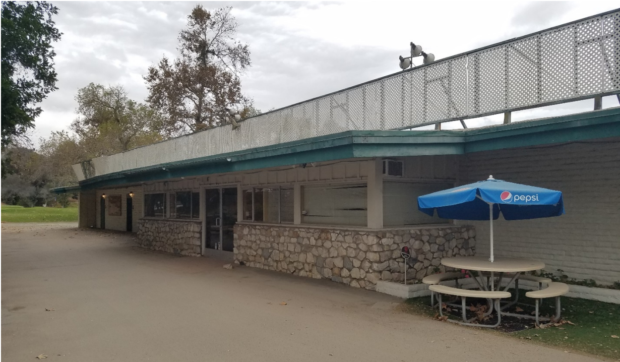
Figure 1. Cottonwood Clubhouse western façade, facing NE (CH-02, 11/19/2019)
