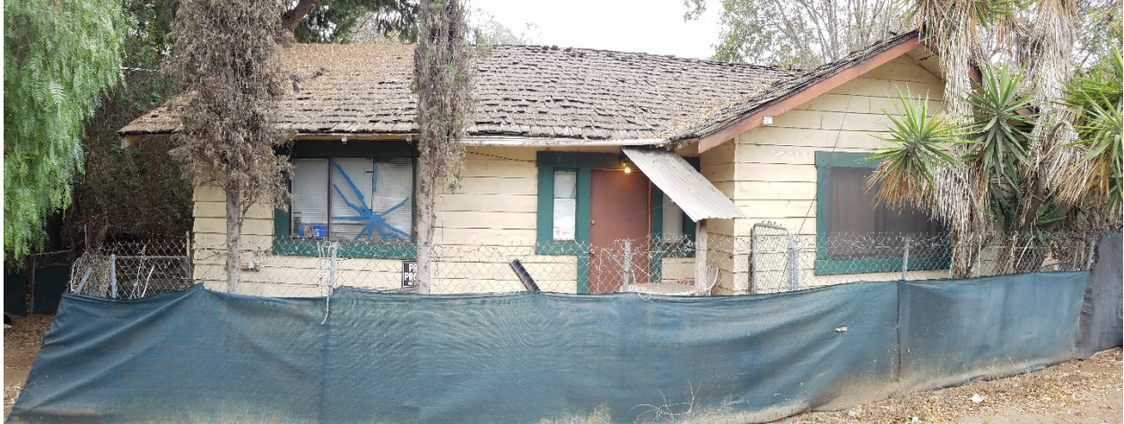
Figure 12. 3629 Willow Glen Drive (P-37-039117) North Façade, facing south (3629-36; 11/19/2019)
