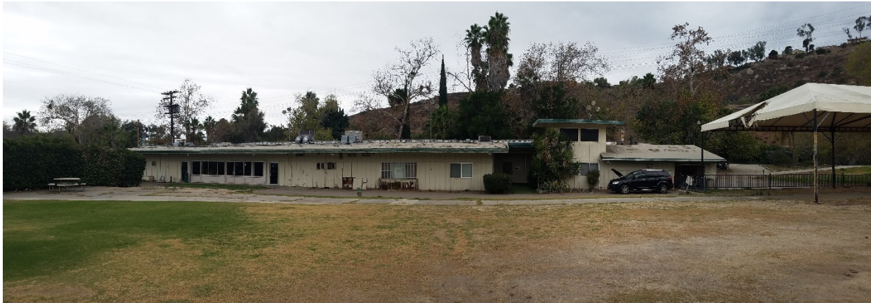
Figure 2. Cottonwood Clubhouse eastern façade, with driving range gazebo at right, facing W (CH-15, 11/19/2019)
