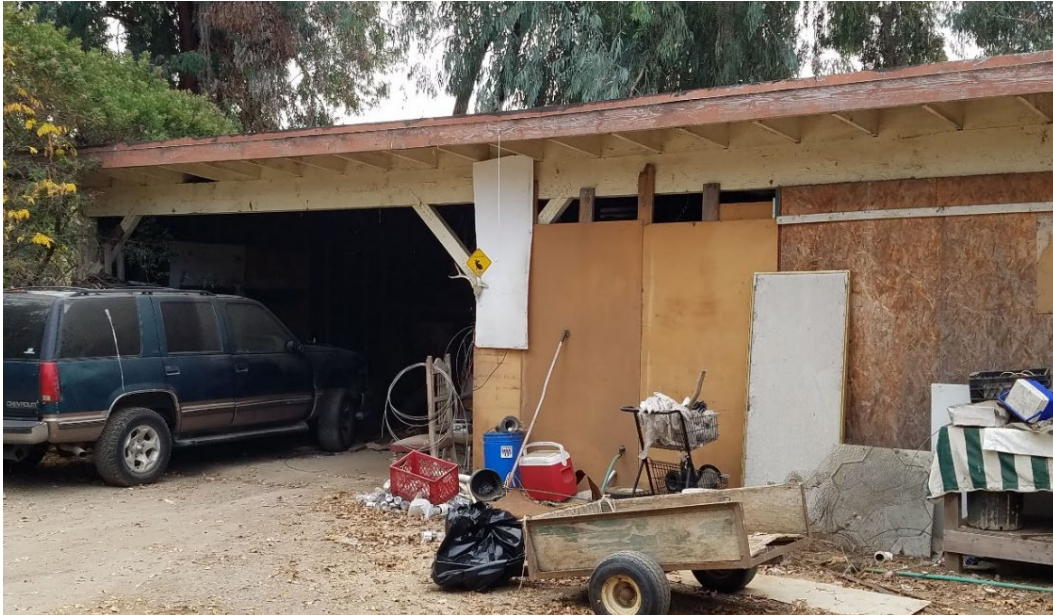
Figure 2. North façade of garage, facing south (3629-17, 11/19/2019).
