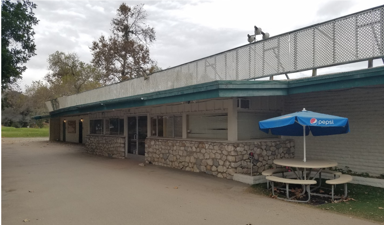
Figure 5. Cottonwood Clubhouse Western Façade, facing northeast (CH-02, 11/19/2019)
