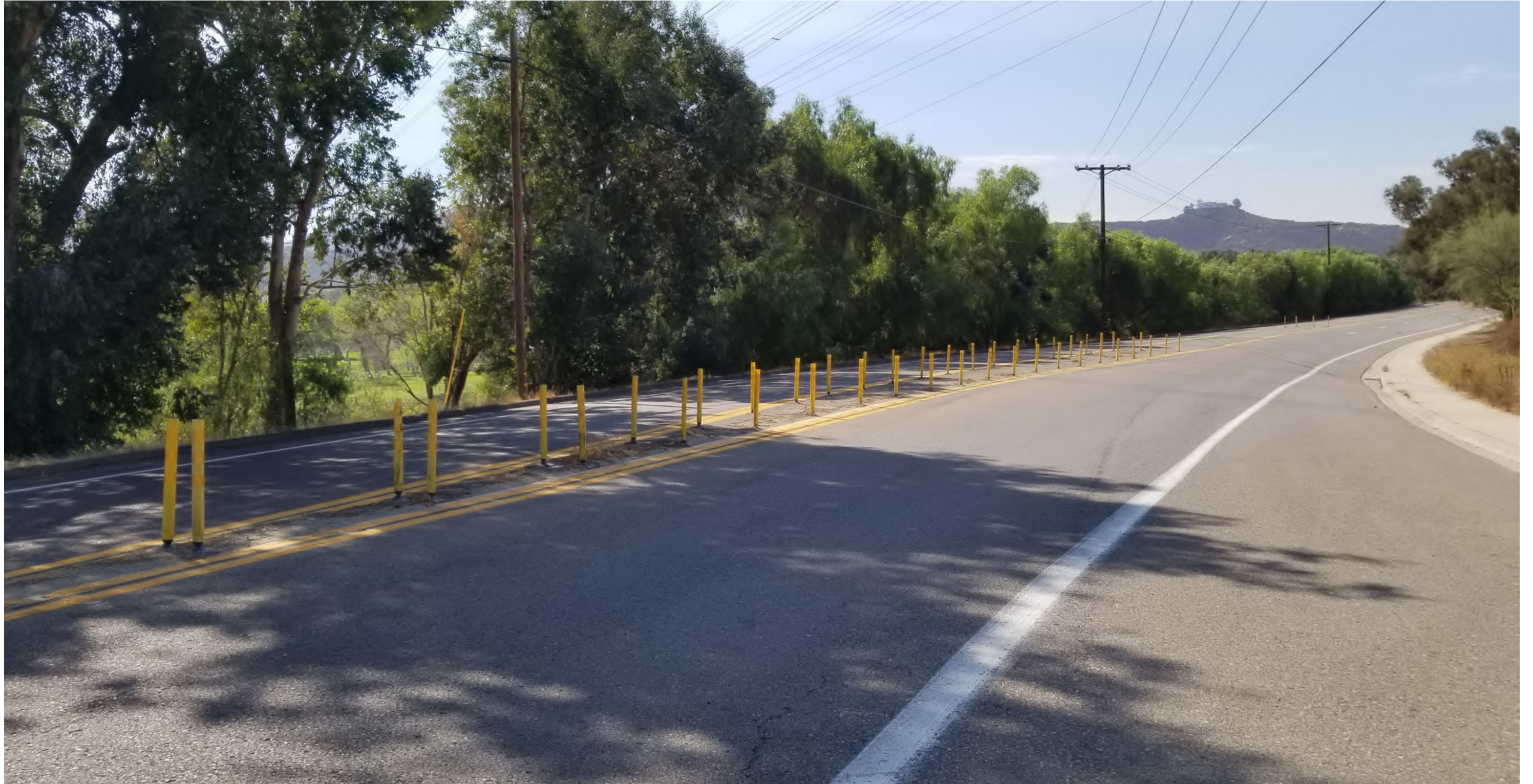
Existing view from Willow Glen Drive towards Project site
