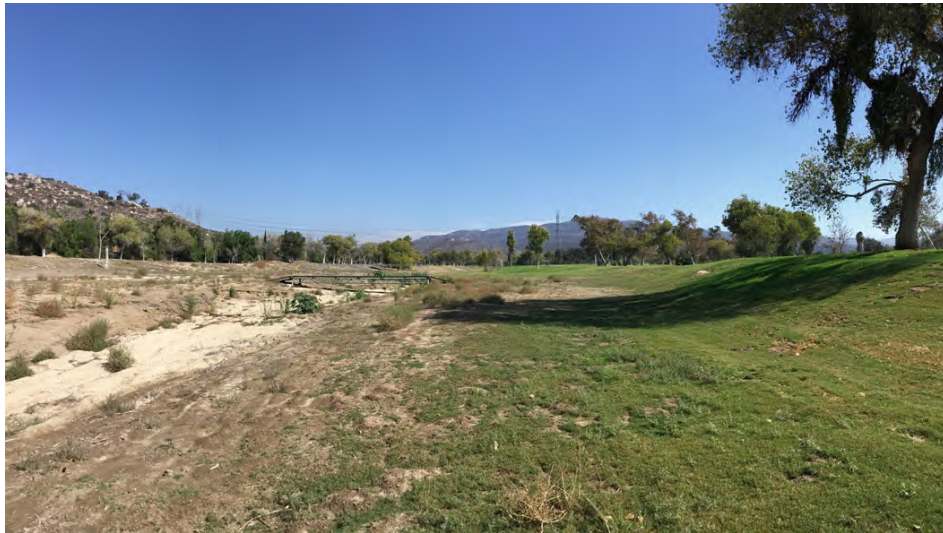
G: Sweetwater River channel looking upstream from east of Steele Canyon Road bridge
