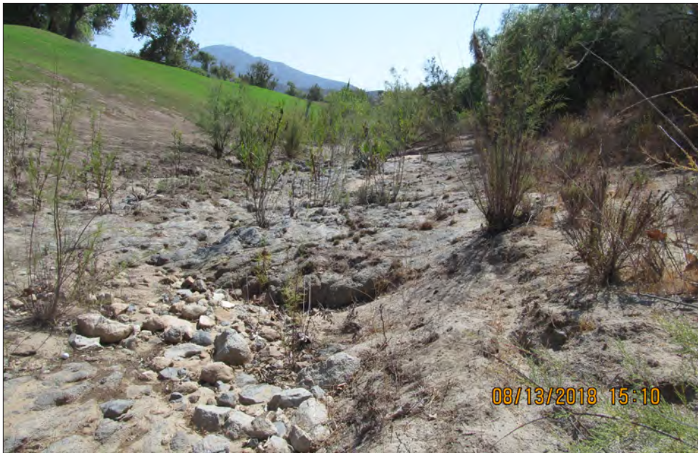
Photo 2. Upstream portion of Sweetwater River where low-flow channel has grouted rock. In northeastern portion of site. Photo is facing southwest (downstream).
