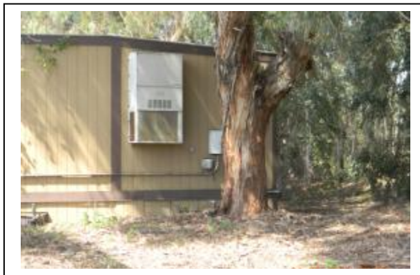
Photos 10 and 11: Any wind driven, ember laden fire in the vicinity of these temporary buildings located in the back of the Adeona Health Care facility will be incinerated from below by flaming wind driven leaf litter, bark fragments and small branch wood (photos by Mike Rogers).
