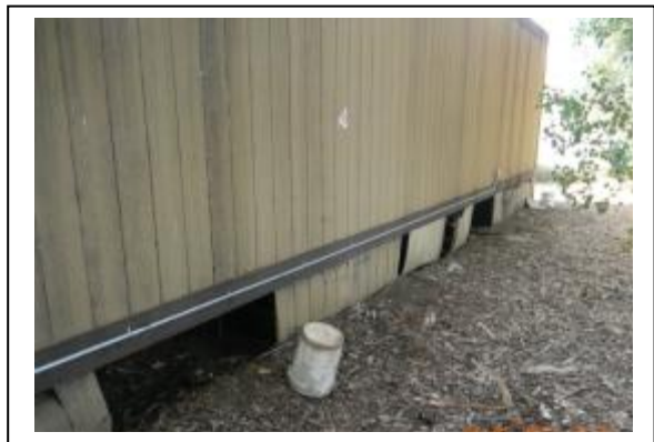
Photos 10 and 11: Any wind driven, ember laden fire in the vicinity of these temporary buildings located in the back of the Adeona Health Care facility will be incinerated from below by flaming wind driven leaf litter, bark fragments and small branch wood (photos by Mike Rogers).
