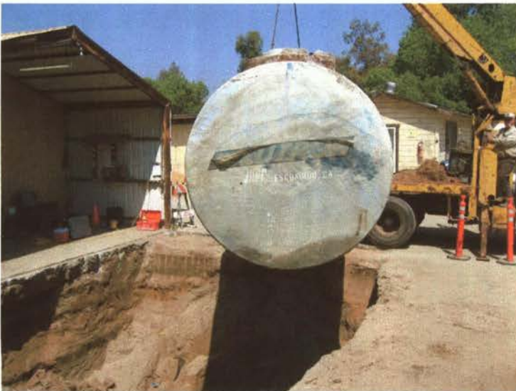
TANK BEING PULED
