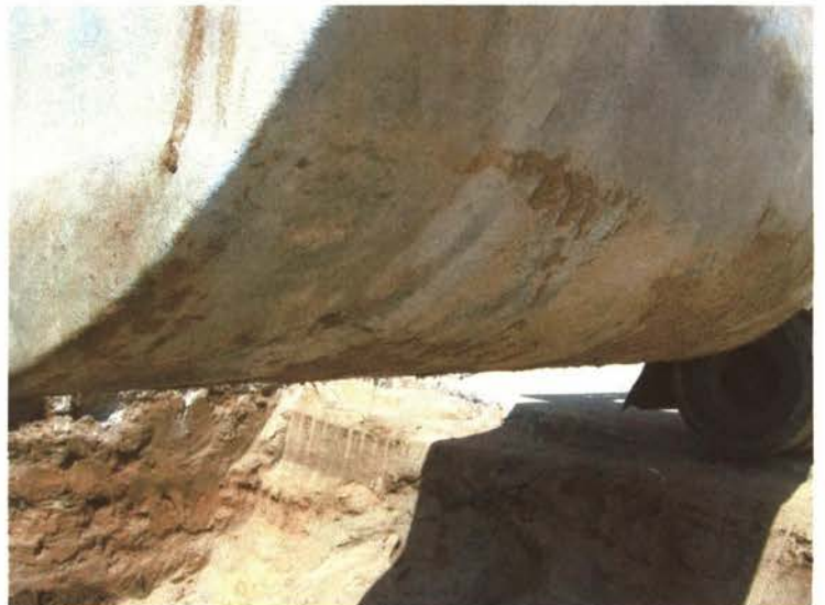
BOTTOM OF TANK
