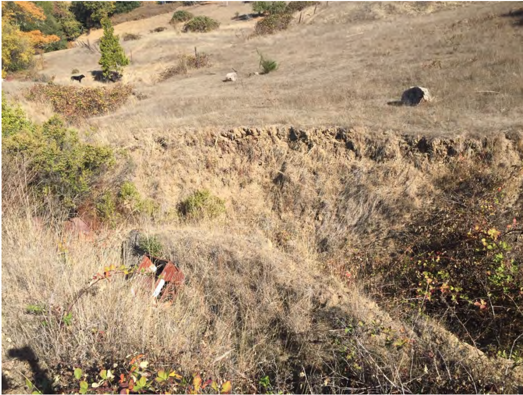
Figure 10. Typical channel incision along east-side tributary. Block-topple in foreground and sloughing on far bank.
