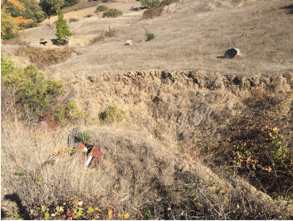
Figure 10. Typical channel incision along east-side tributary. Block-topple in foreground and sloughing on far bank.
