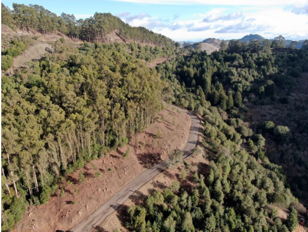
This picture of the Claremont Ave project was taken from the west. Photo by Doug Prose, Courtesy Hills Conservation Network.
