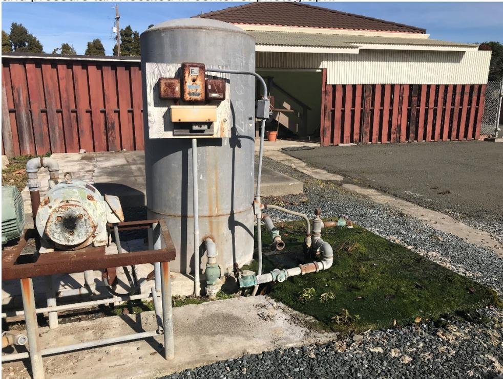
Photograph 4. Water well and pressure tank. Water was observed seeping from wellhead causing vegetation growth.
