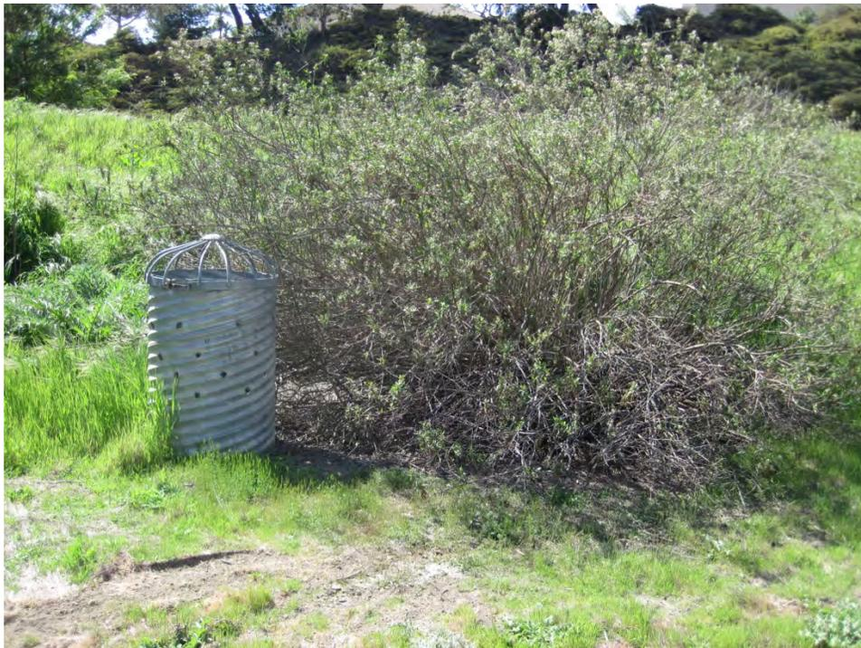
Photo 10. View of the standpipe at the west end of the swale which appears to transmit storm water to storm drain system.
