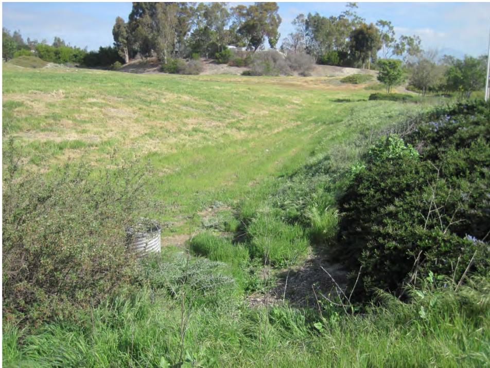
Photo 8. View of the swale which appears to collect storm water sheet flowing over study area to prevent it from running into parking lots and buildings (standpipe in foreground).
