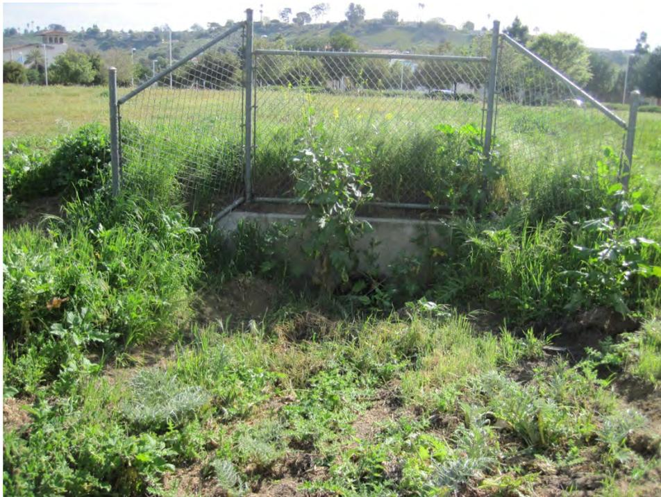
Photo 4. View of concrete inlet which appears to collect runoff from adjacent manufactured/landscaped slopes between the study area and residential development.
