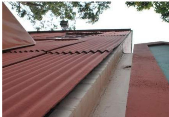
Figure 26: Transition between Building 2 (brick and corrugated metal) and Building 1.
