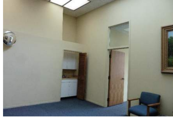
Figure 42: Interior view of office spaces in Building 3.
