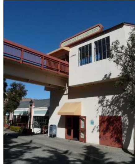
Figure 46: Two-story enclosed stairwell connecting the pedestrian skybridge to Building 1.
