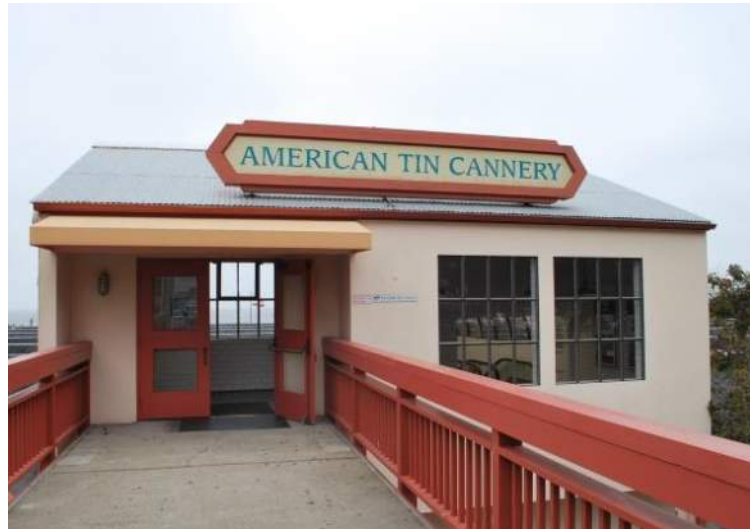
Figure 48: Second story entrance to enclosed stairwell via skybridge. View looking northeast.
