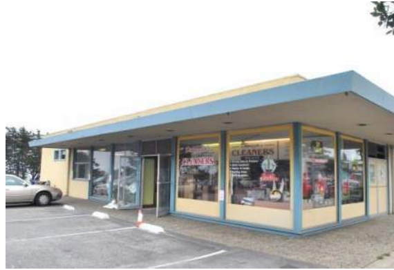
Figure 54: 124 Central Avenue, Di Maggio's Classic Cleaners.
