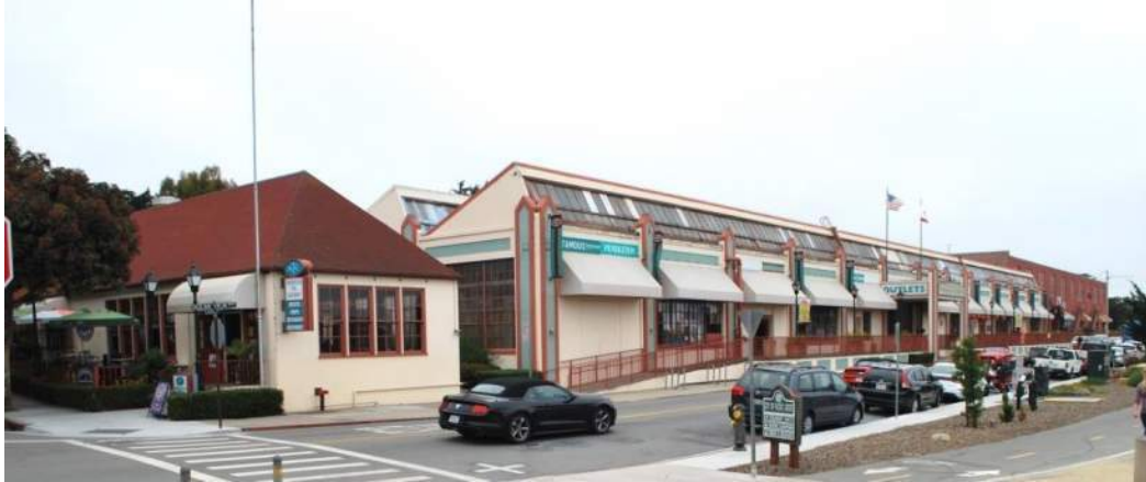
Figure 2: Northeast façade. Building 0 at left, Building 1 at middle, Building 2 at right. Building 3 at far right is recessed and not visible. View facing northwest.
