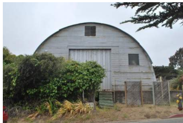
Figure 58: Quonset hut at 119 Dewey Avenue, across from Building 3.
