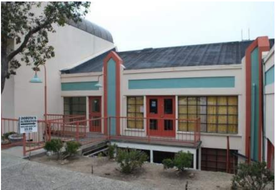
Figure 19: Southwest façade of Building 1, right of the skybridge.
