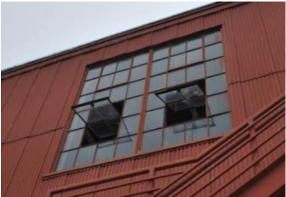
Figure 27: Industrial steel windows with four-lite pivot sashes at Building 2.
