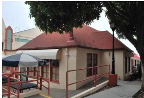
Figure 11: Partial view of the southwest (left) and southeast (right) façades of Building 0, looking north.
