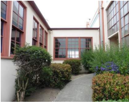
Figure 9: Connecting corridor between Building 0 (left) and Building 1 (right), looking southwest.
