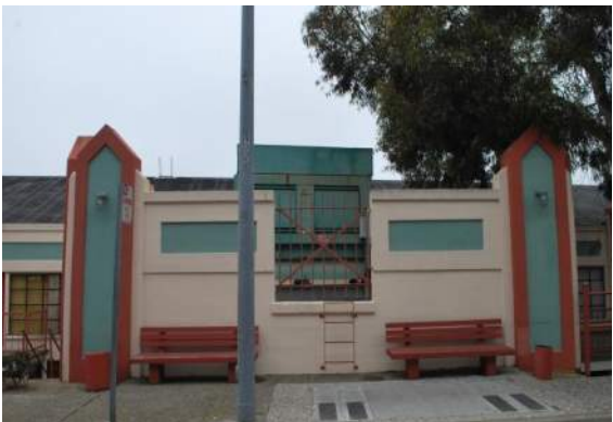
Figure 21: Projecting bay on the southwest façade, framed by chevron capped concrete piers.
