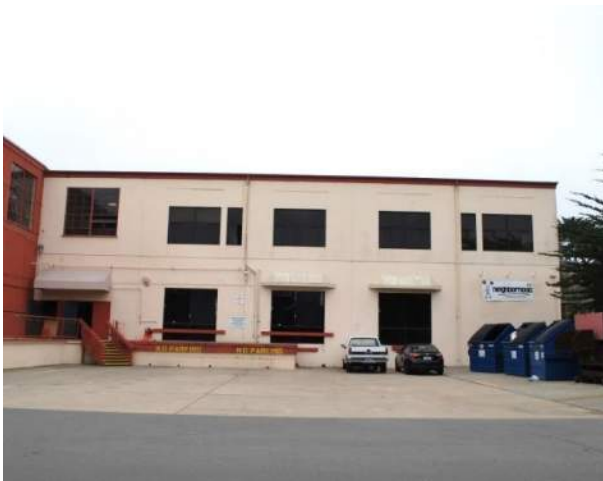
Figure 32: Building 3 primary (northeast) facade, looking southwest.
