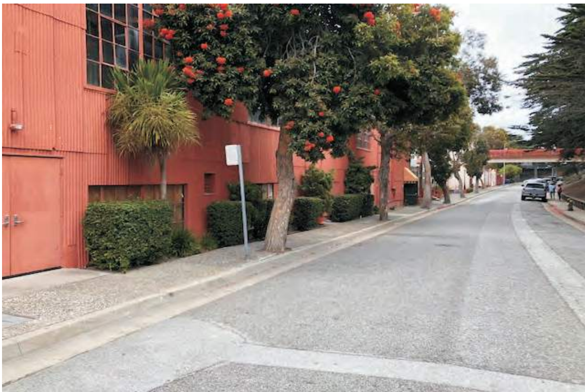
Photo 5: View along Sloat Avenue; elevated walkway in background.
