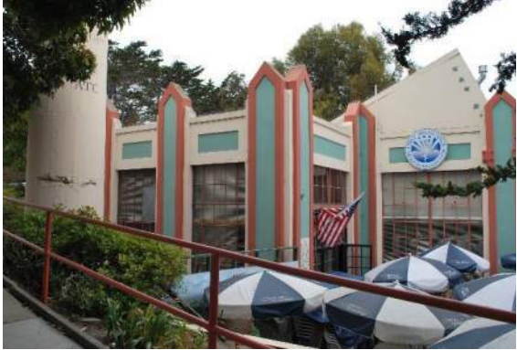
Figure 23: Projecting flat roof mass at the southwest corner of Building 1, and the concrete smokestack, looking west.
