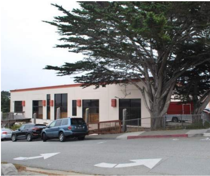
Figure 36: Building 3 northwest façade. The second story is visible from Dewey Avenue.
