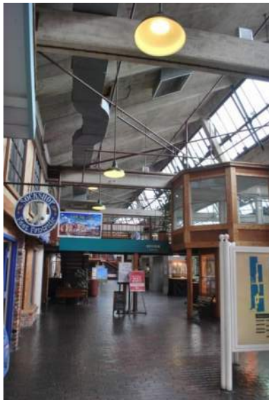
Figure 39: Interior view of Building 1, including sawtooth clerestory windows and double-height space with mezzanine level.
