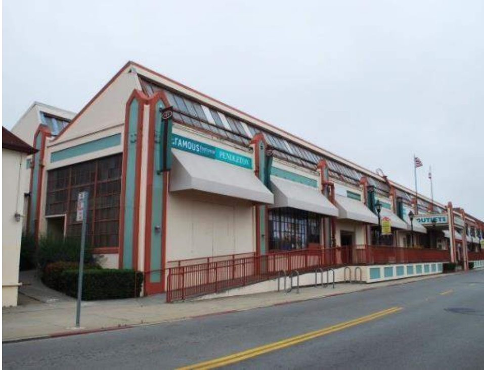
Figure 12: Primary façade (right) and southeast façade (left) of Building 1 with storefronts and elevated promenade, looking northwest. Typical northeast facing sawtooth clerestory windows are visible.
