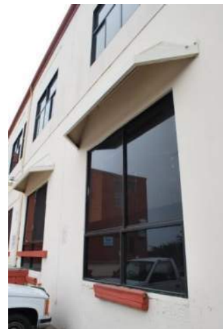
Figure 33: Building 3 fixed first story windows.
