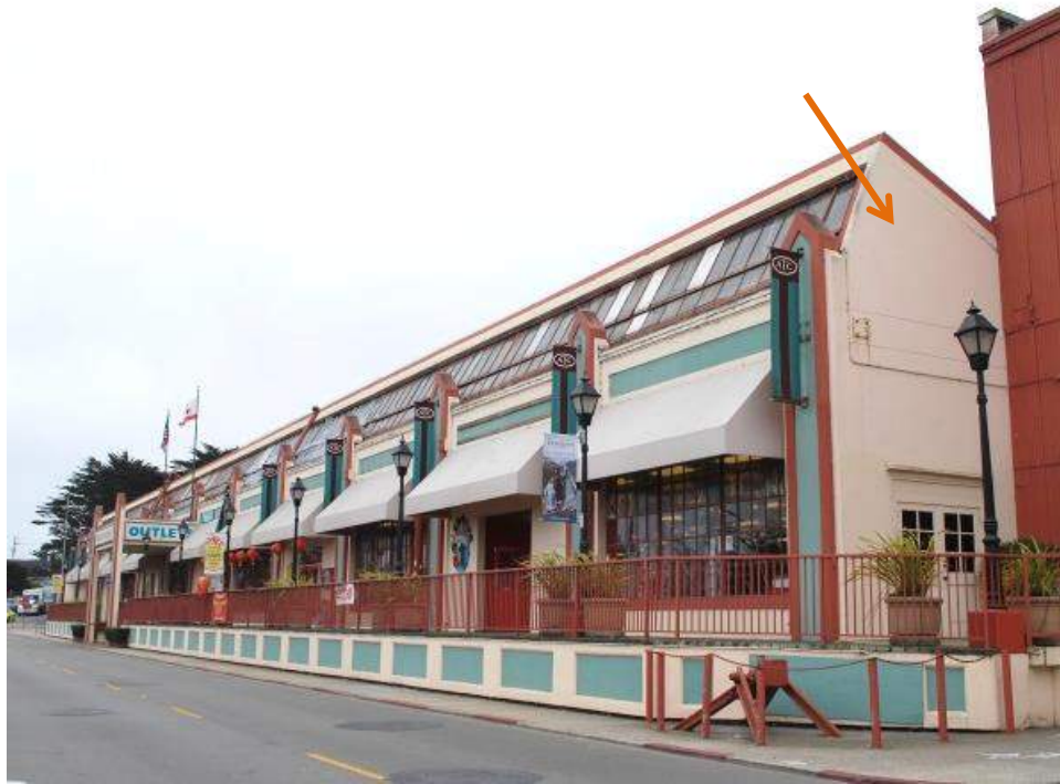
Figure 15: Primary (southeast) façade of Building 1 (left), the exposed portion of the northwest (right, indicated by orange arrow), and Building 2 (far right). View facing south.
