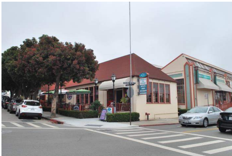
Figure 3: Building 0 southeast façade (left) and northeast façade (right), looking west.
