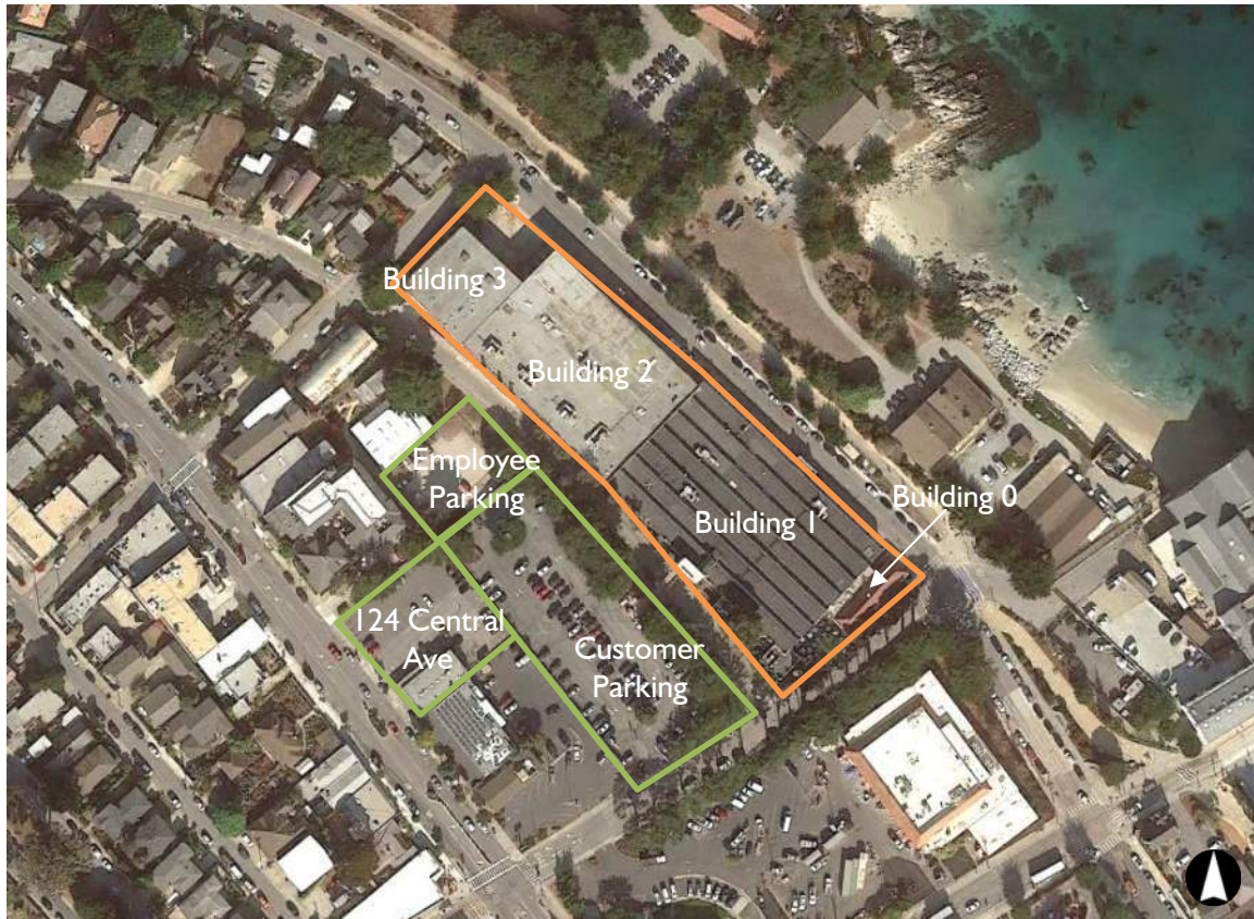
Figure 1: 109/125 Ocean View Boulevard (APN 006-231-001), outlined in orange. The adjacent customer parking lot (APN 006-234-005), employee parking lot (APN 006-234-005), and 124 Central Ave (APN 006-234-008), are outlined in green. Source: Google Earth Pro, November 2018. Edited by Page & Turnbull.
