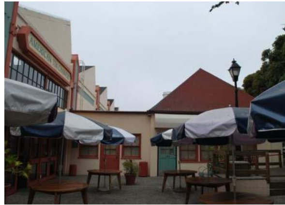
Figure 10: Southwest façade of Building 0, looking northeast.
