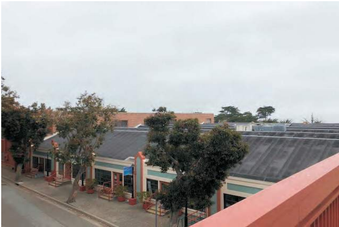
Photo 10: View across Building 2 roof towards Building 1 from walkway.
