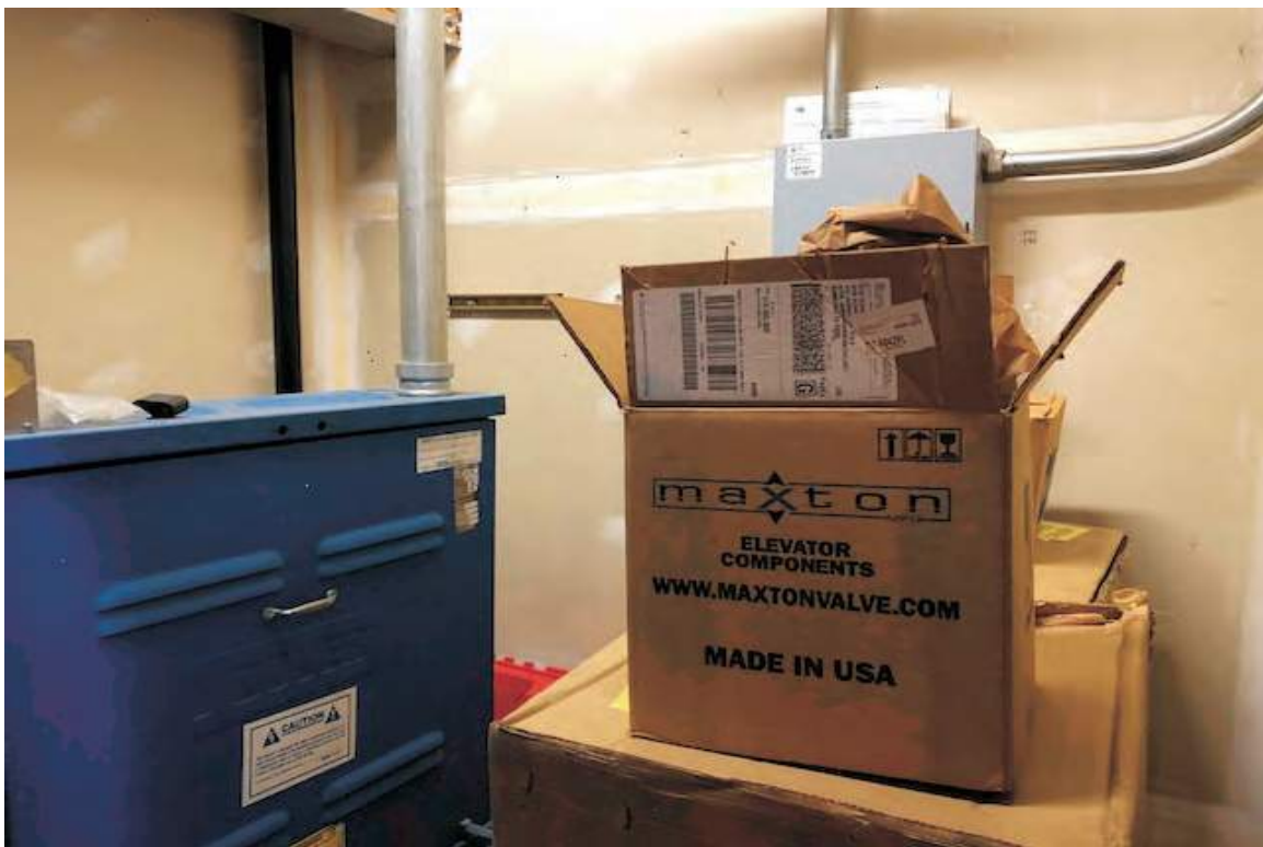
Photo 23: Elevator equipment room.
