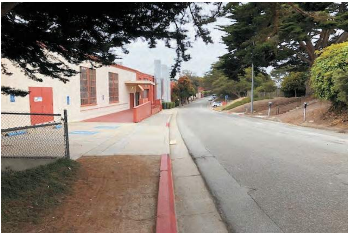
Photo 13: View south along Building 3 exterior along Dewey Street.
