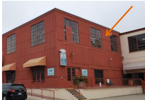
Figure 28: Northwest façade of Building 2, view looking south.
