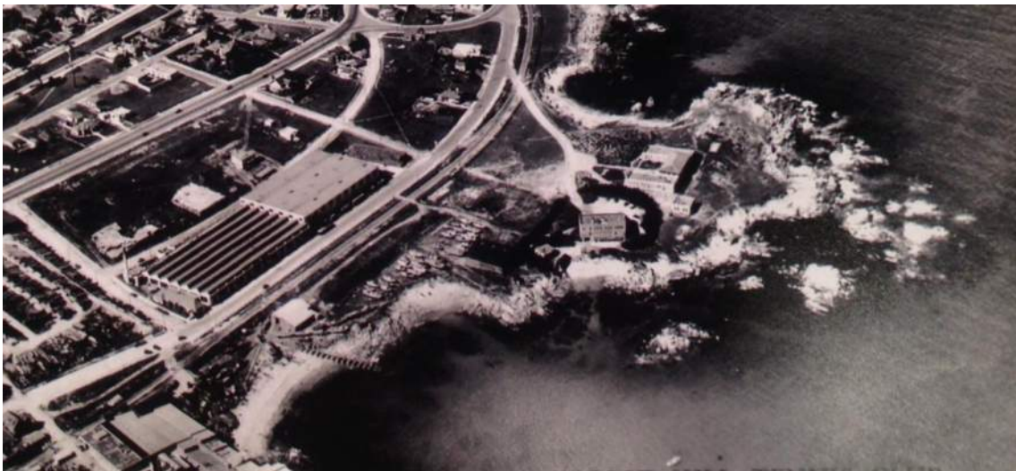
Figure 63: Bird's-eye view of the American Can Company (Buildings 0, 1 and 2), 1932. Source: Mr. Pat Hathaway California Views Historical Photo Collection, CV# 86-085-0033.
