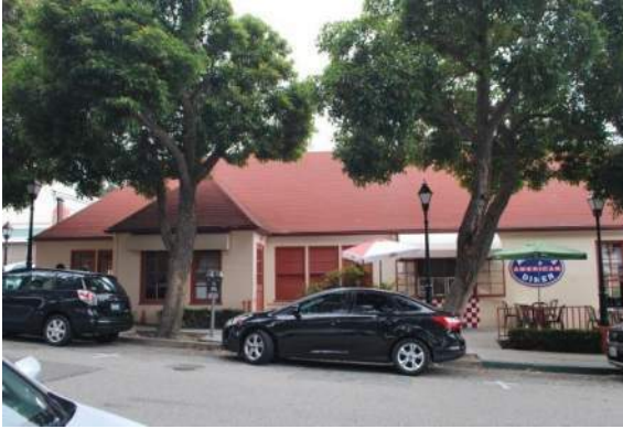
Figure 4: South (left) end of the southeast façade of Building 0, looking northwest.
