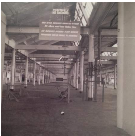
Figure 69: Interior view of vacated Building 1, 1972. Source: Mr. Pat Hathaway California Views Historical Photo Collection.
