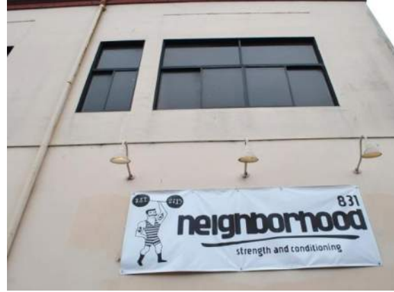
Figure 35: Building 3 second story fixed and sliding windows.
