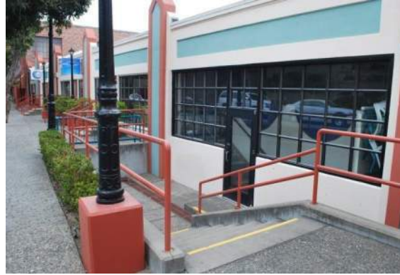
Figure 18: Partial view of southwest façade of Building 1, left (north) of skybridge, looking northwest.
