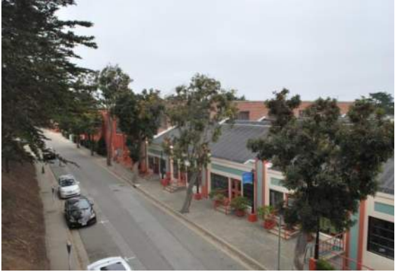
Figure 17: Partial view of Building 1 southwest façade from the skybridge, looking northwest.
