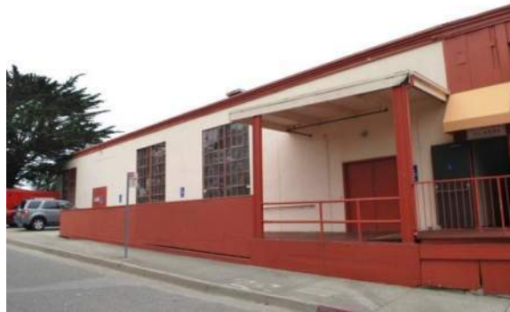
Figure 38: Building 3 southwest façade, looking northeast.
