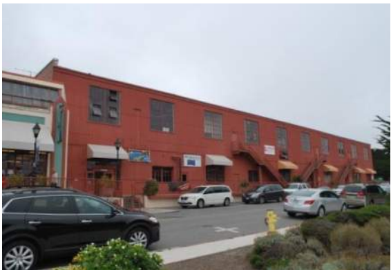
Figure 25: Primary (southeast) façade of Building 2, facing west.
