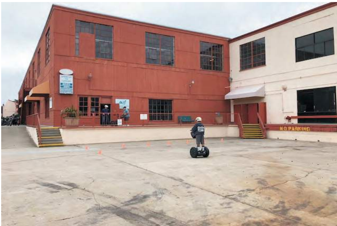
Photo 11: Former loading area adjacent to Buildings 2 and 3.
