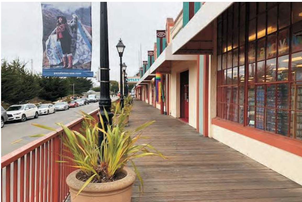
Photo 2: ATC exterior looking south along Ocean View Boulevard.
