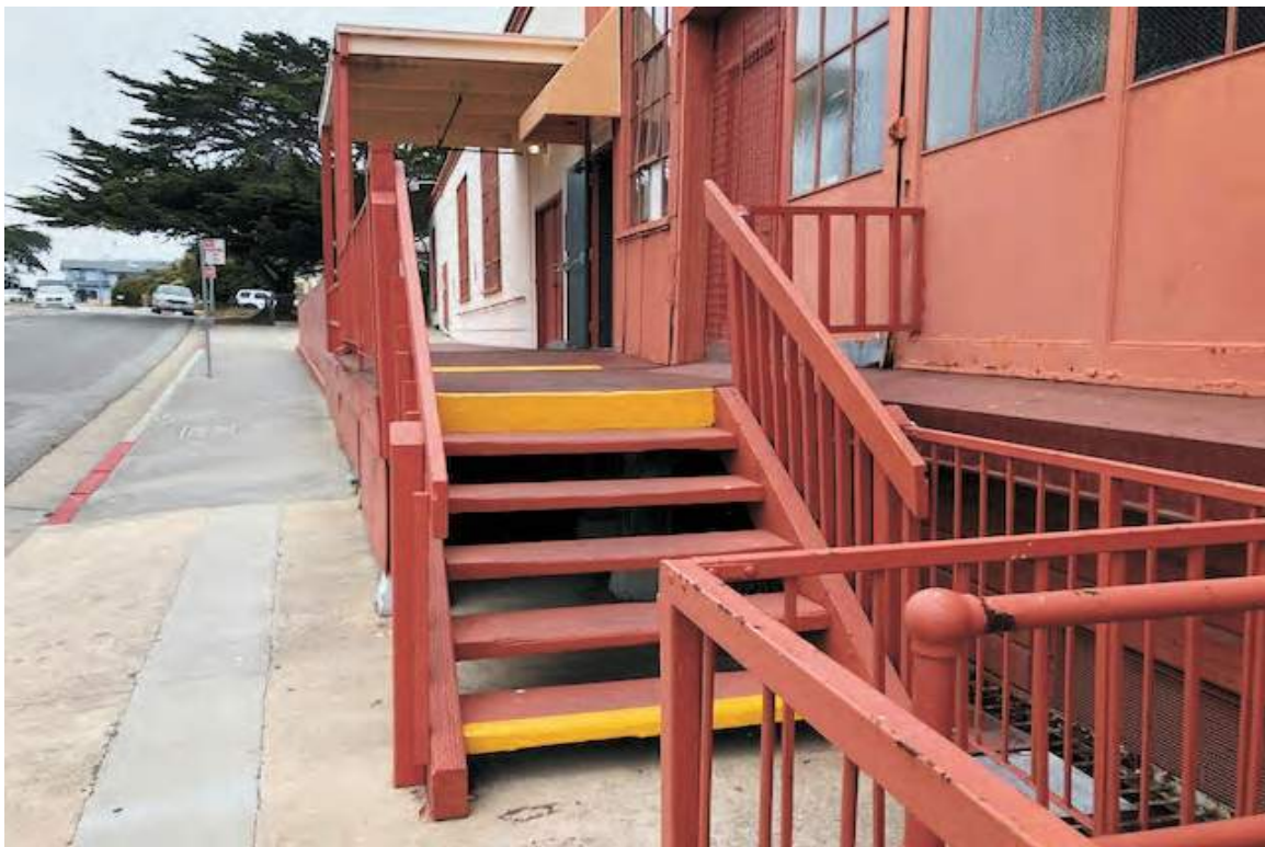
Photo 6: Sloat Avenue exterior; view west towards Dewey Street.
