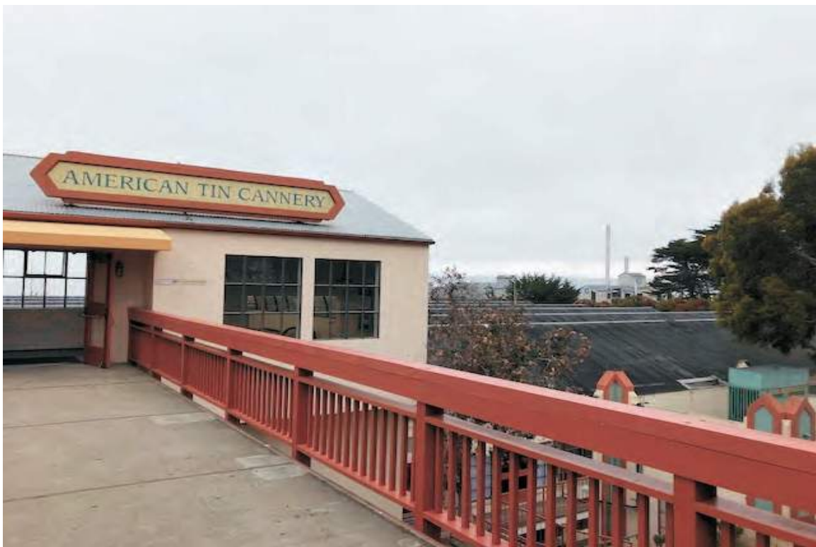
Photo 9: View from walkway across Building 1 roofline.
