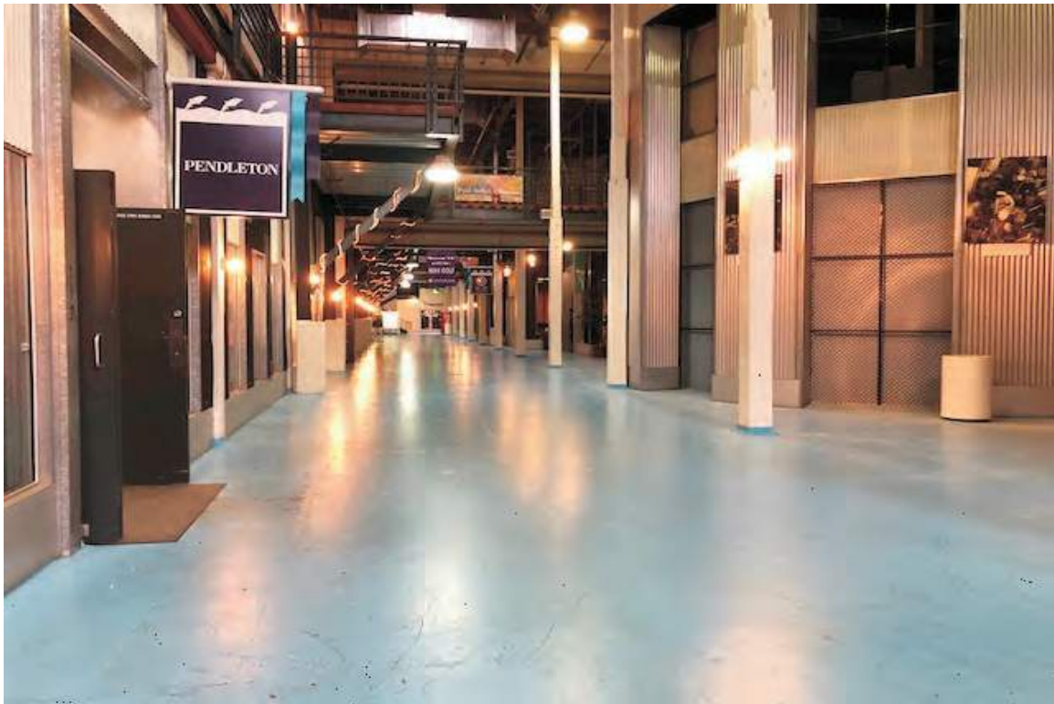
Photo 15: Interior of Building 2, view towards Building 1.
