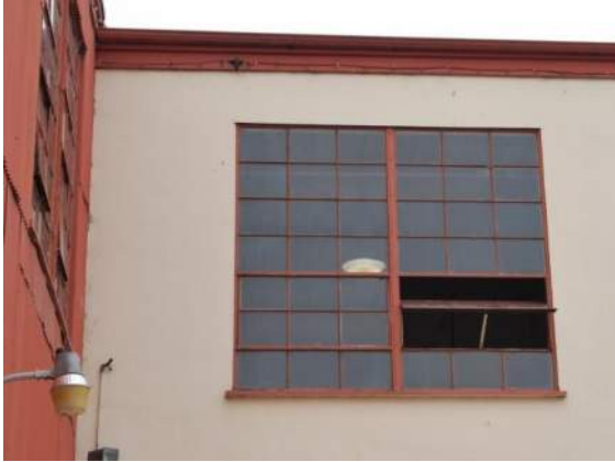
Figure 34: Building 3 second story warehouse window with six-lite pivot sashes.
