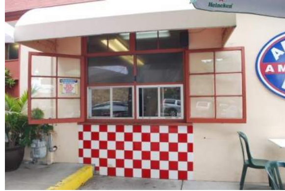
Figure 5: Paired casement window with transom on the southeast façade.
