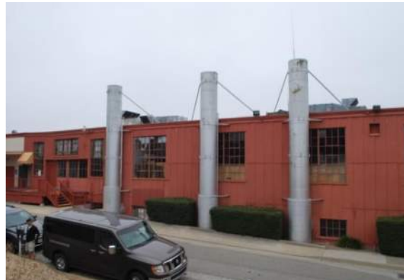
Figure 30: Building 2 southwest façade, looking northeast.
