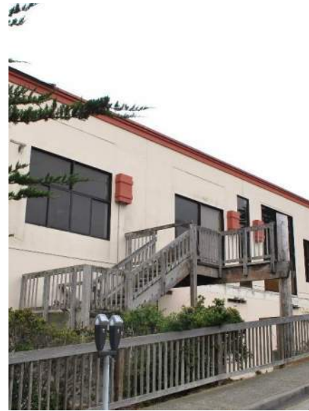
Figure 37: Exterior stair at far left (north) of Building 3 northwest façade.
