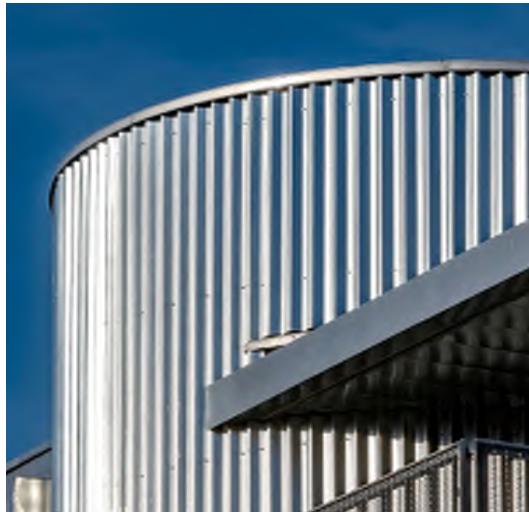
Vertical Painted Corrugated Metal Siding
