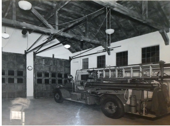
Figure 16: 3917 Apparatus room, looking northwest, date unknown. (courtesy, Station No. 9)
