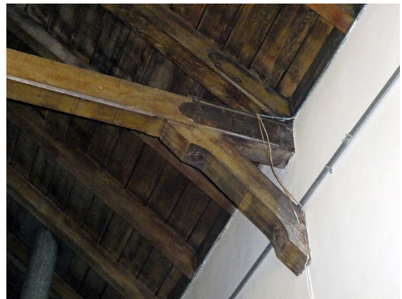
Figure 30: Detail of wood truss ceiling in apparatus room (GPA, 2019)
