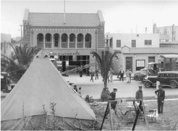
Figure 21: Station No. 9 was considered unsafe immediately after the earthquake and small tents were used as living quarters, 1933 (Goodrich, 83)
