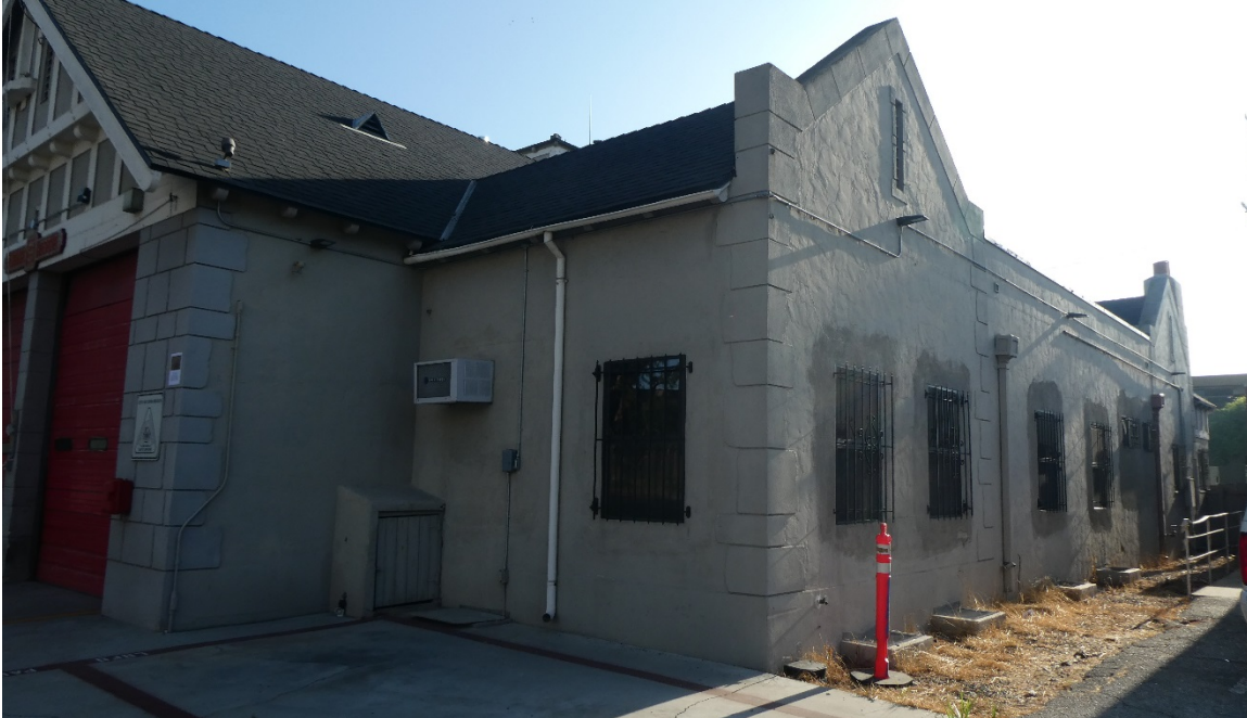
Figure 7: South elevation, view looking northeast (GPA, 2019)
