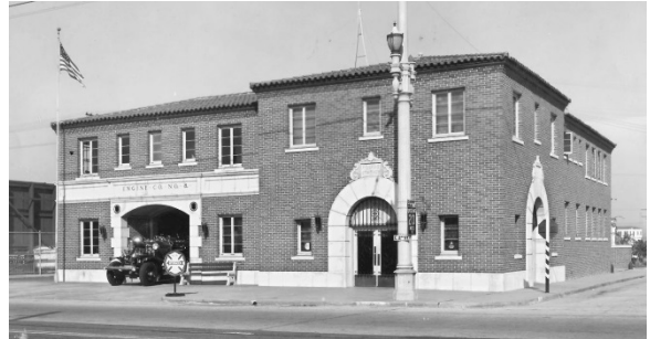
Figure 25: Station No. 8 was constructed in 1929 as a typical urban, two-story fire station, date unknown (Goodrich, 149)
