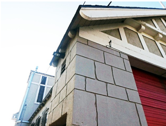
Figure 29: Detail of faux ashlar exterior finish, view of northwest corner (GPA, 2019)
