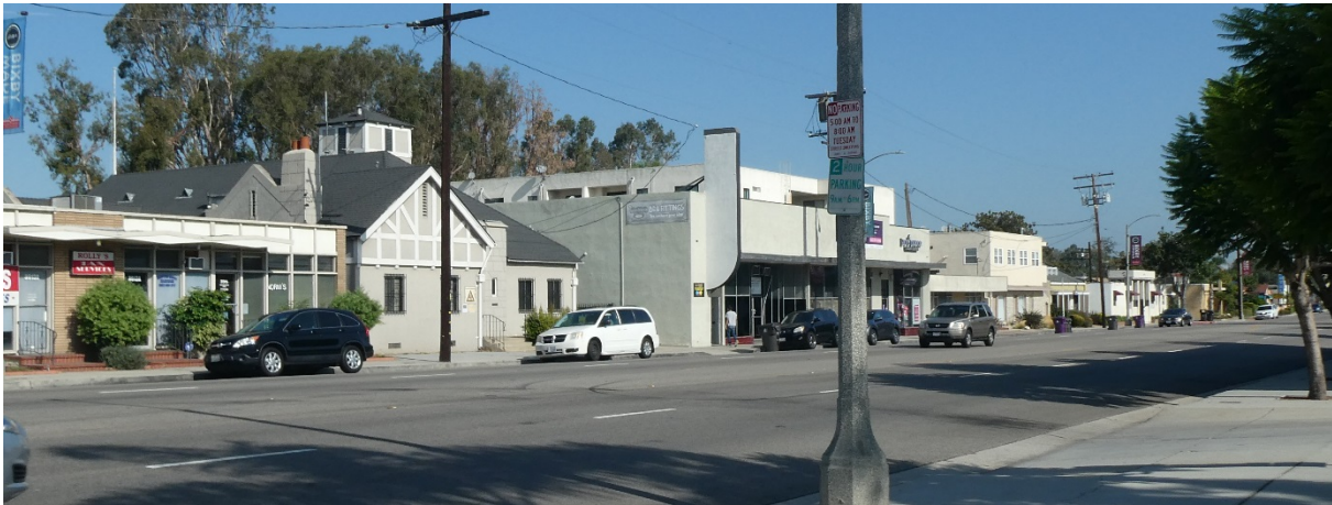
Figure 2: 3917 Long Beach Boulevard, looking northwest (GPA, 2019)
