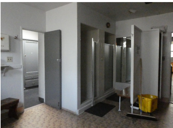
Figure 13: Wash rooms, looking north (GPA, 2019)
