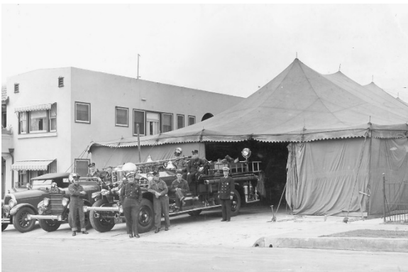
Figure 23: After demolition, a Barnum Circus tent was erected onsite of Station No. 9, date unknown (Goodrich, 86)
