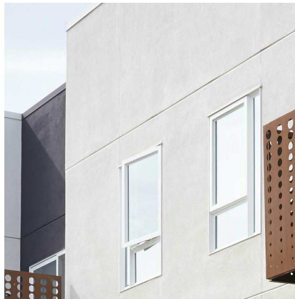
CEMENT PLASTER, WHITE ALTERNATE TYPICAL CLADDING MATERIAL
