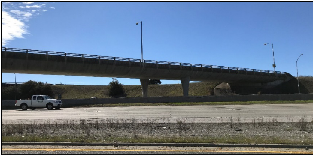
Photo 7: Sand Hill Road OC (South and North); View south east of Sand Hill Road OC North Bridge (Bent 2 and Abutment 1)
