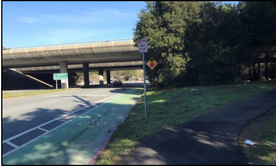
Photo 10: Alpine Road UC (L/R) Bridges; View eastbound of designated bike path and Alpine Trail
