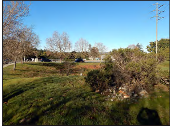
Photograph 2. Overview of the Project Area showing utility box (facing west).
