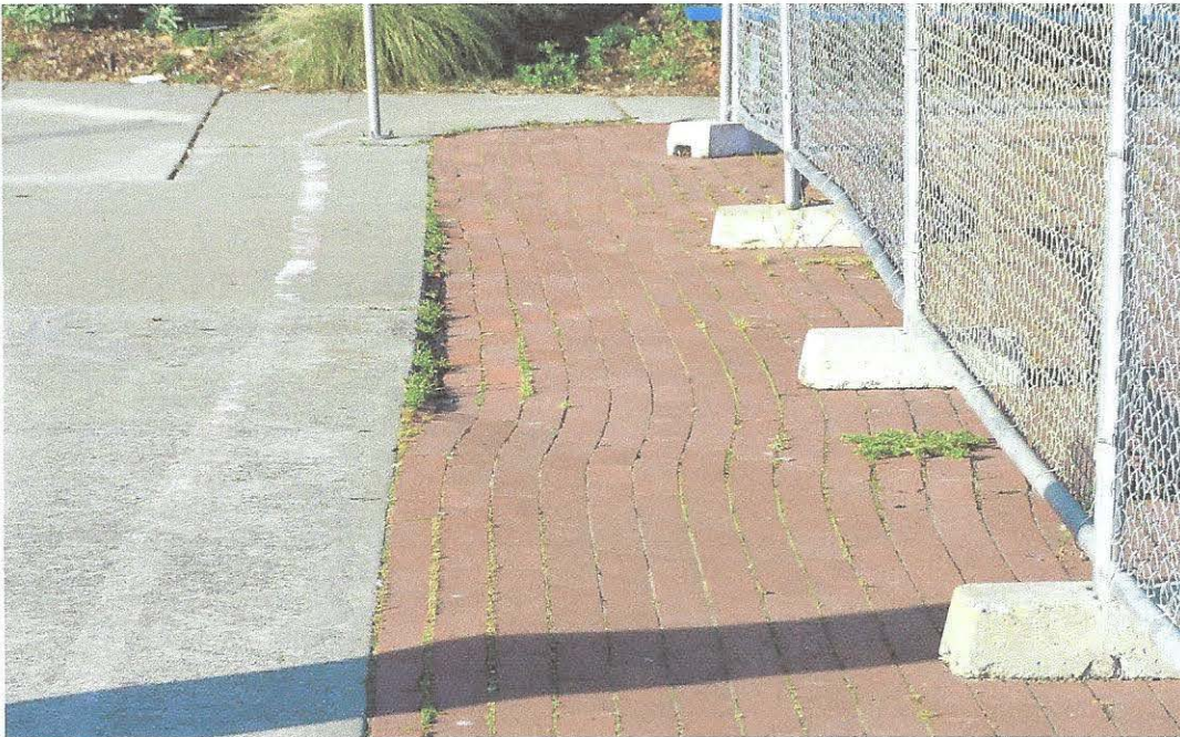
The Hayward fault causes visible disruption of the ground at Contra Costa Community College, as shown in this photograph of displaced bricks on the campus:
