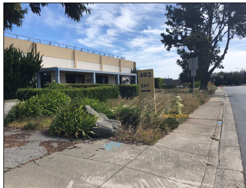
SITE APPROACH FROM WEST
