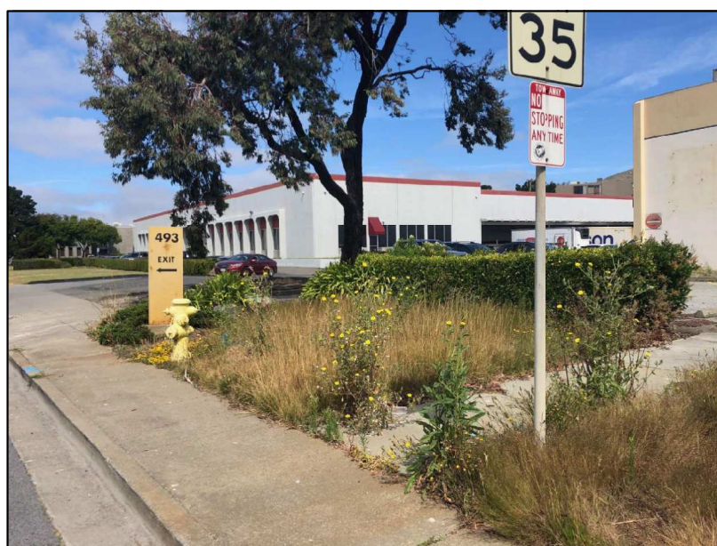
ADJACENT WEST BUILDING
