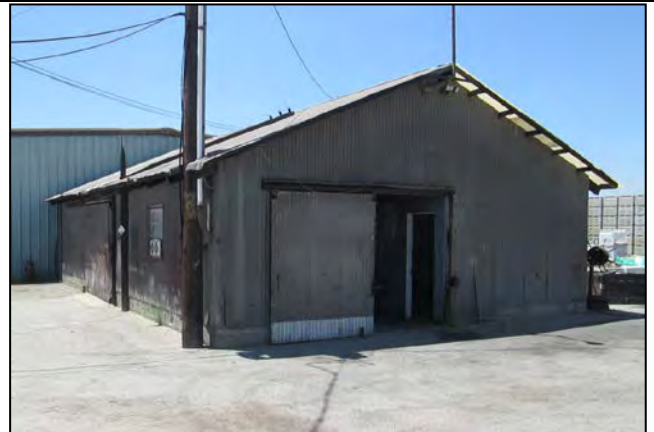
Former Maintenance shop building. View looking south.
