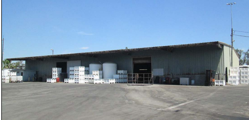
Figure 14: Vegetable processing building, view looking northwest.
