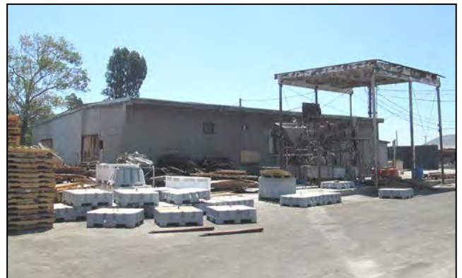
Former packaging and dicing building, view looking southeast.
