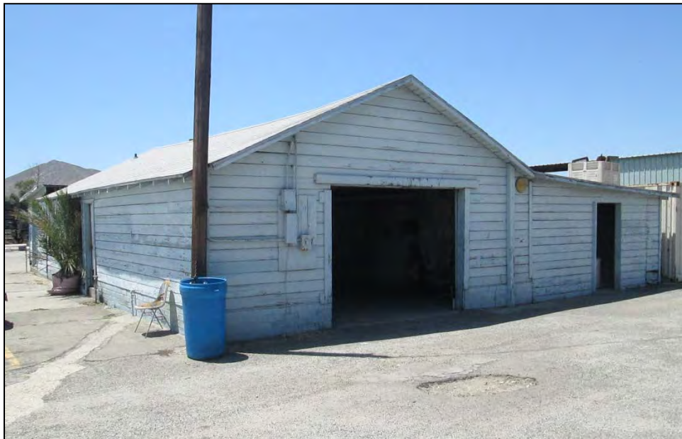
Figure 12: Storage and office building. View looking southwest.
