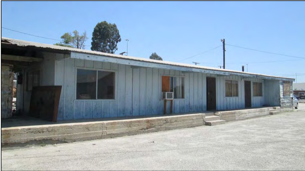
Figure 10: South elevation of office building, now vacant. View looking northeast.
