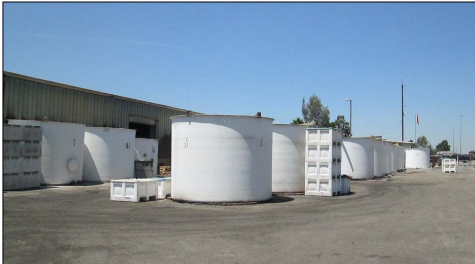
Figure 15: Brining vats located on the north side of the vegetable processing building. View looking west.
