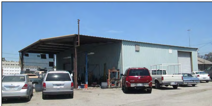
Figure 17: New maintenance building, view looking northwest.
