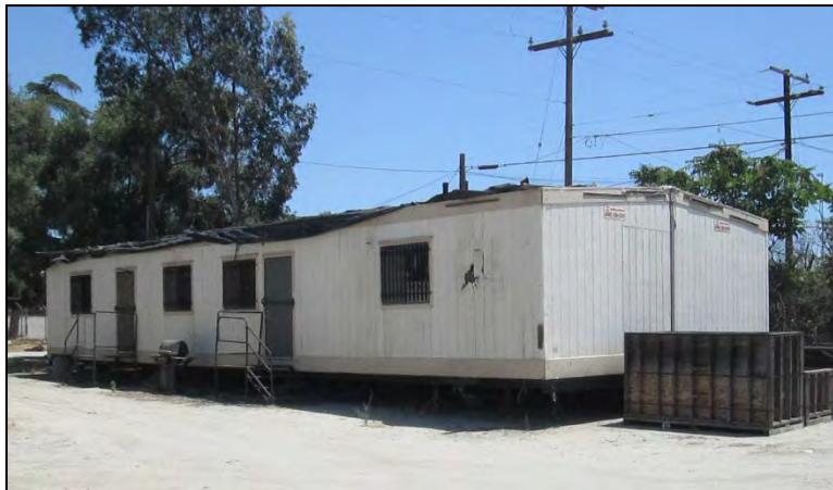
Figure 18: Double-wide manufactured office unit, view looking northeast.
