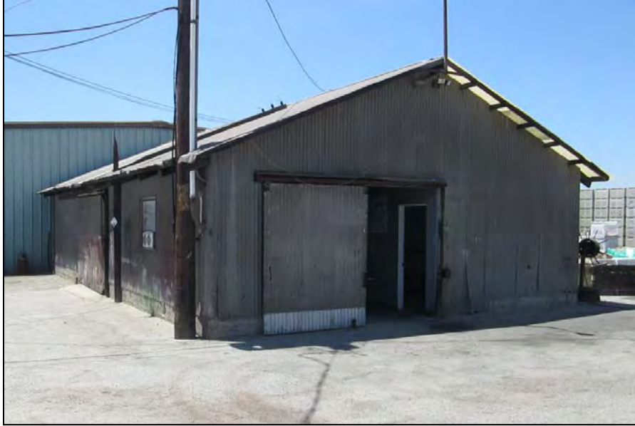
Figure 11: Former Maintenance shop building. View looking south.
