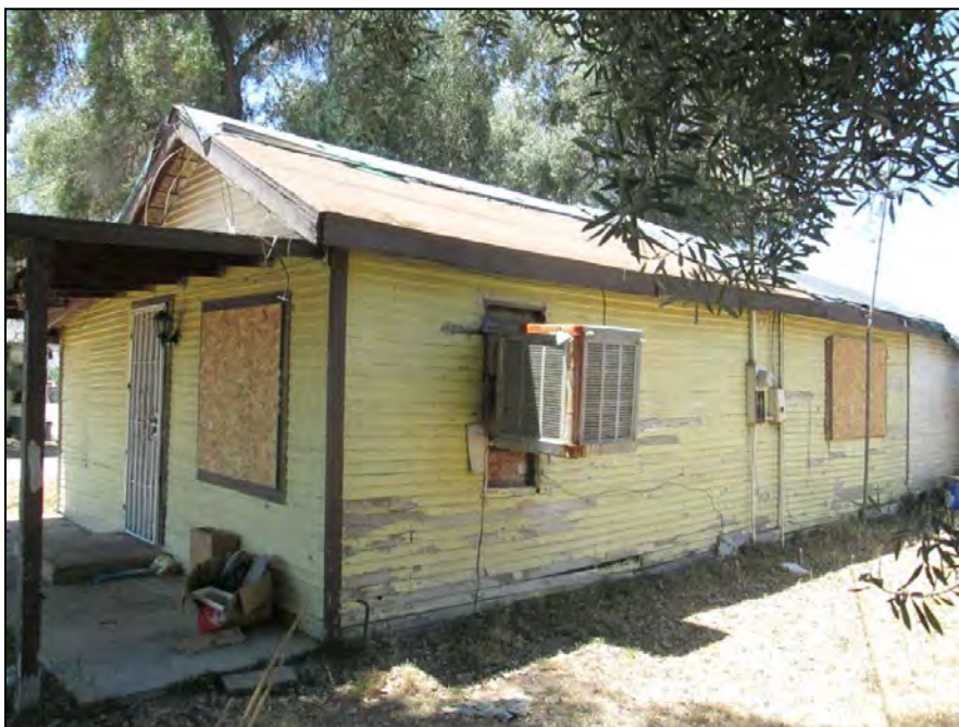
Figure 8: East (front) and north elevation of dwelling. View looking southwest.
