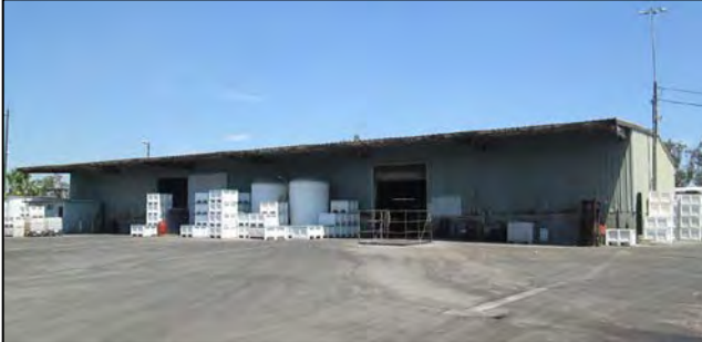
Vegetable processing building, view looking northwest.
