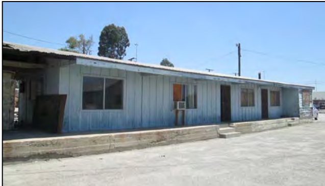
Former office building, now vacant. View looking northeast.
