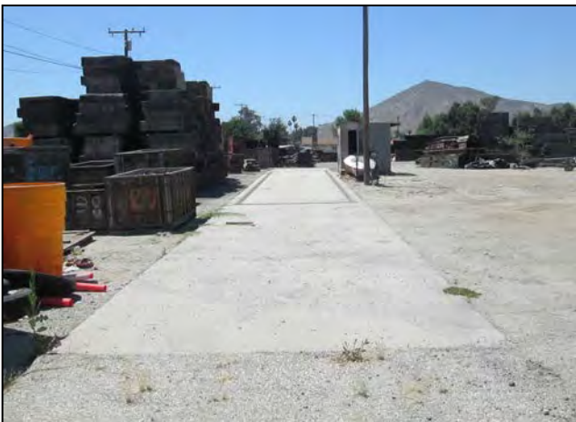
Truck scale and attendant hut, view looking south.
