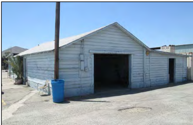
Storage and office building. View looking southwest.
