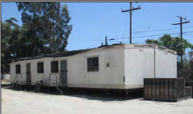
Storage and office building. View looking southwest.
