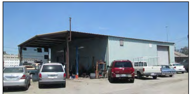
New maintenance building, view looking northwest.
