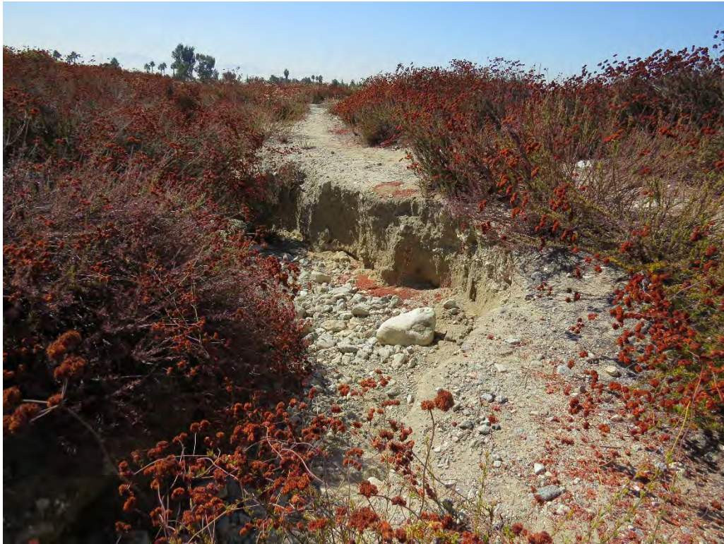
Photograph 23: Looking at the middle of Drainage 3 where it becomes more incised as it slopes down the hill on the site.
