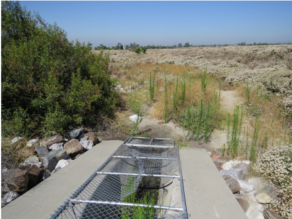
Photograph 9: Looking west over the outflowing culvert.
