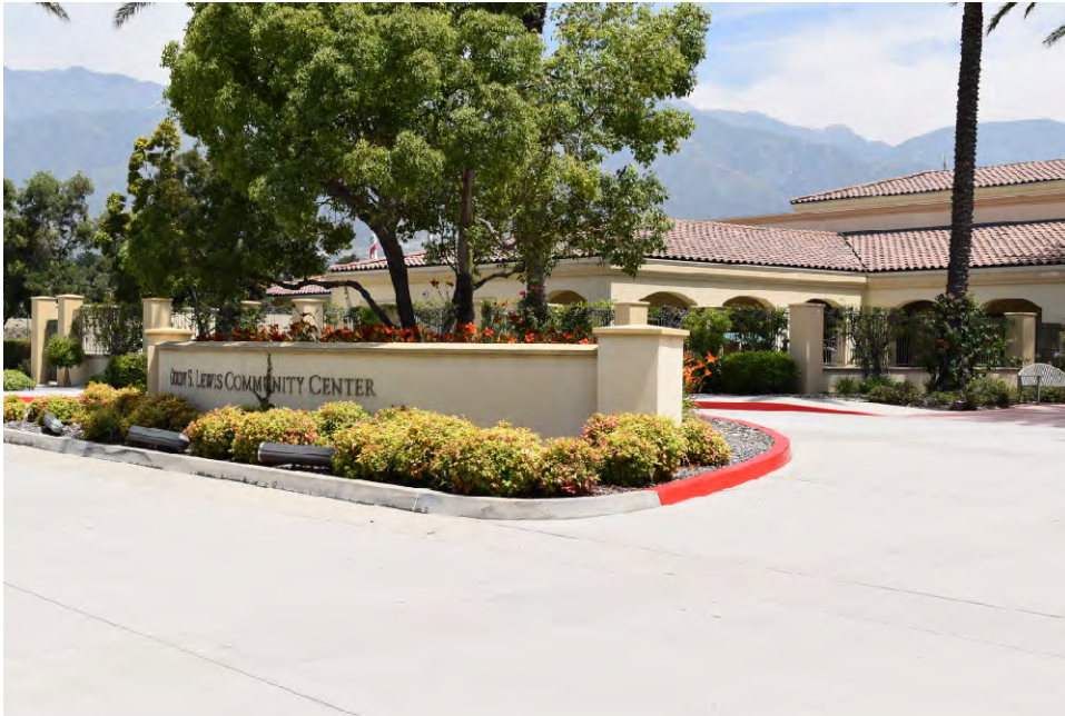
Goldy S. Lewis Community Center, southwest side of the joint facility building.
