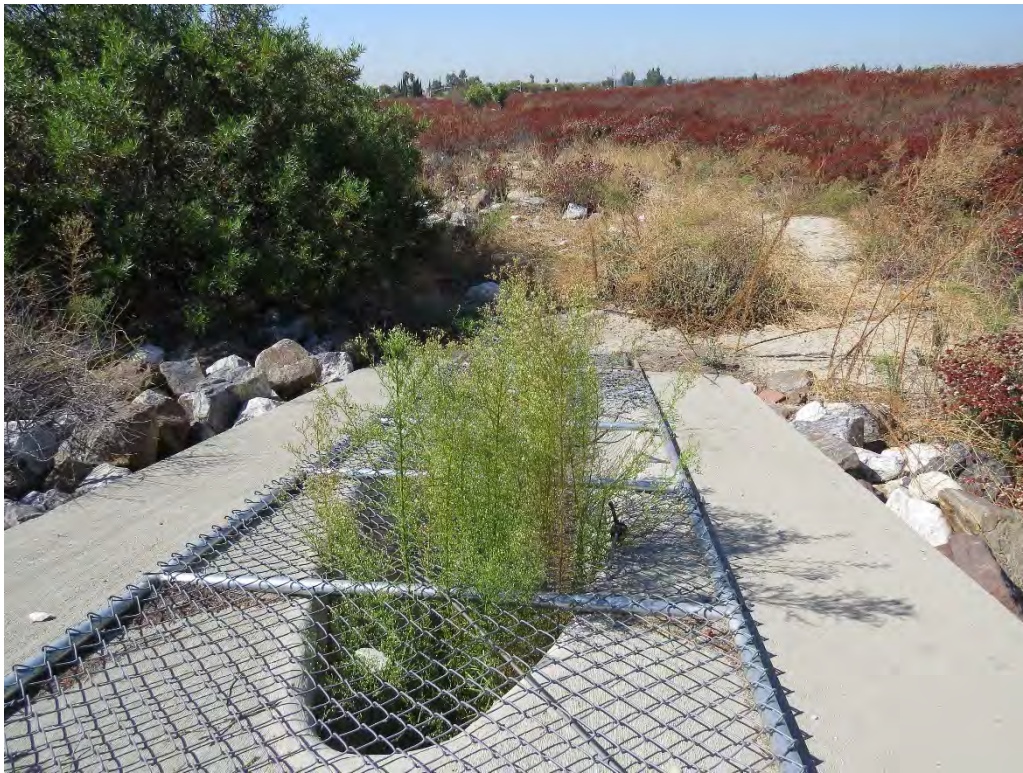
Photograph 1: Looking west at the beginning of Drainage 1.
