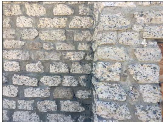
Fig 1 (left): Subject property, west elevation (center) and south façade (right), view northeast (McGee, 2019); Fig 2 (right): Subject property, west elevation, detail of concrete rubble exterior wall material, view west (McGee, 2019)
