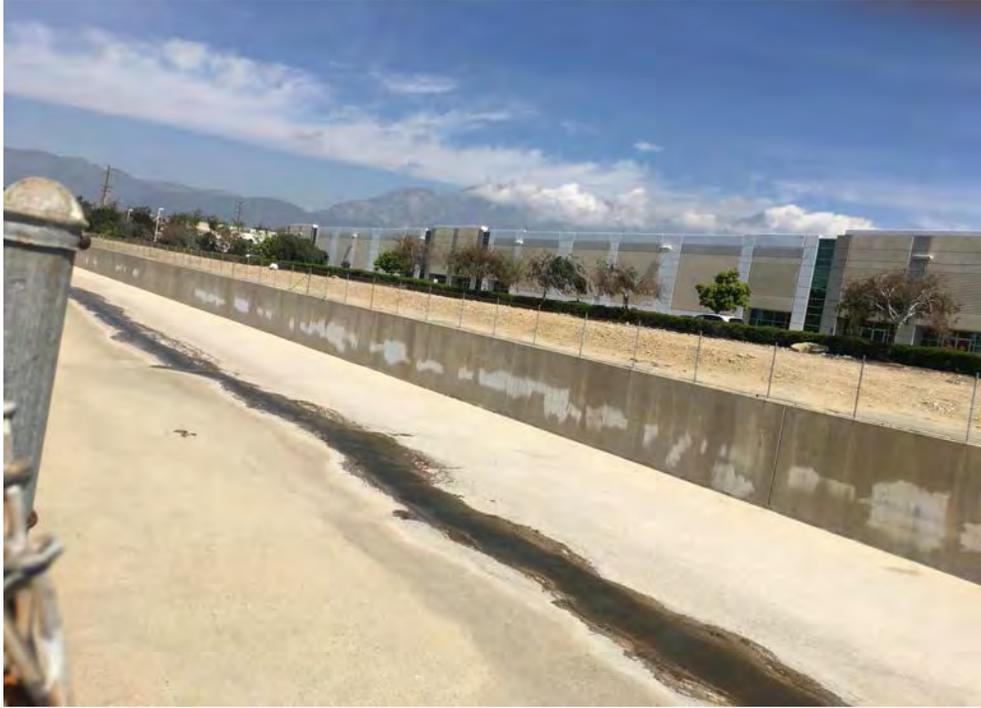
Photo 7. Upstream view of Ordinary High Water Mark data point 1 (OHWM 1) taken within the concrete-lined Cucamonga Creek located just east of the project boundary and survey area. Ten-foot wide low-flow channel estimated by presence of flowing water and staining. 76-foot wide active floodplain estimated based on the flat channel bottom and 5- and 10-year flow events that occur within the full extent of the channel.
