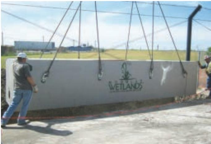
The MWS Linear is simple, easy to install, and has a space-efficient design that offers lower excavation and installation costs compared to traditional tree-box type systems. The structure of the system resembles precast catch basin or utility vaults and is installed in a similar fashion.
