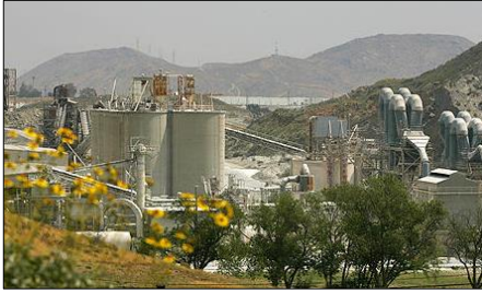
Figure 6-8: Former Riverside Cement Company plant, Jurupa Valley
