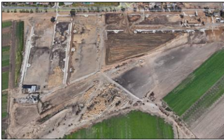
Figure 5-2: Subdivision under construction, Jurupa Valley
