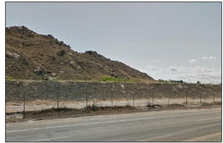
Figure 8-21: Flood levee along Santa Ana River in Jurupa Valley
