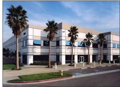
Figure 11-5: Logistics building, Jurupa Valley
