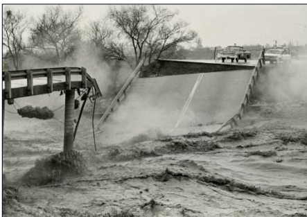
Figure 8-7: Van Buren Bridge collapse during the 1969 Santa Ana River flood (Riverside County Flood Control and Water Conservation District)
