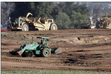
Figure 7-11: Construction graders, Inland Empire
