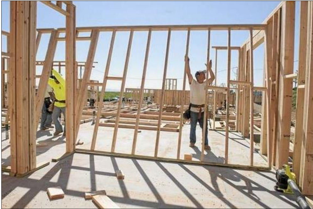
Figure 5-1: New housing construction in Jurupa Valley
