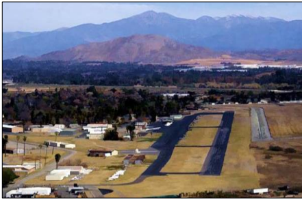
Figure 2-30: Historic Flabob Airport
