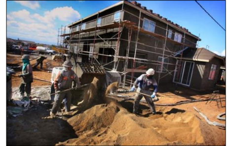
Figure 11-4: New housing under construction near Vernola Marketplace
