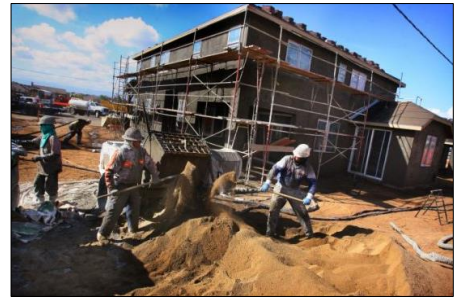
Figure 5-4: Housing construction in Jurupa Valley
