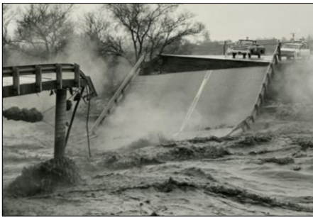
Figure 4-12: Van Buren Bridge collapse during 1969 Santa Ana River flooding
