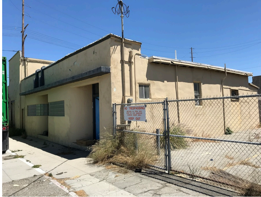
Figure 10-3. Nakamura Multi-Use Building, primary (west) elevation and south elevation, camera facing northwest.
