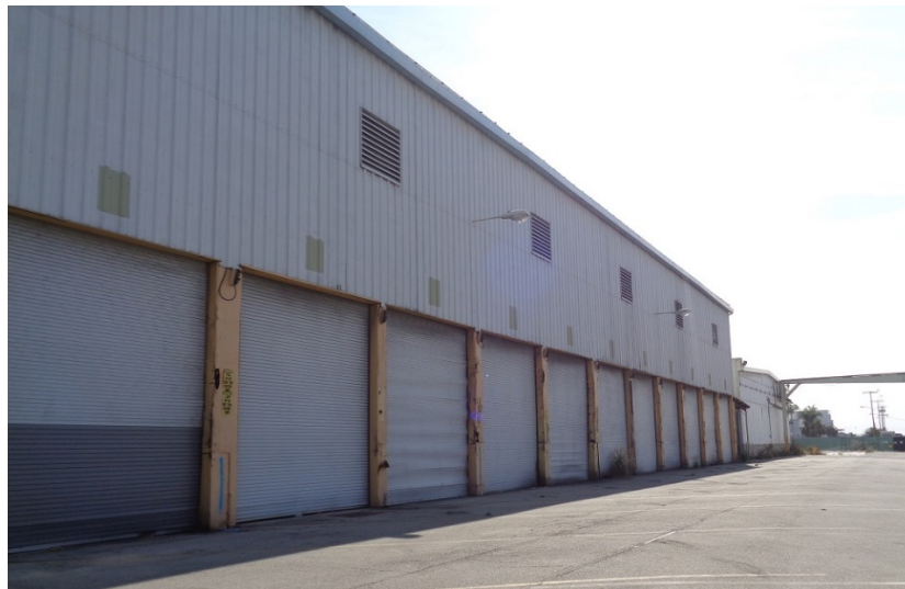
Figure 5-38. West elevation, Warehouse portion of facility in foreground (left) and Cold Storage portion in the distance (right), camera facing south.
