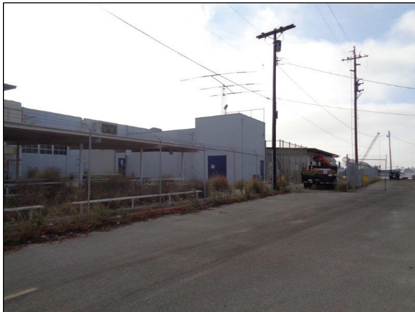
Figure 12: Star-Kist Plant No. 4, primary (west) elevation, overview of southwest corner of Plant No. 4 (volumes 7-9), camera facing southeast. ICF, 2018.
