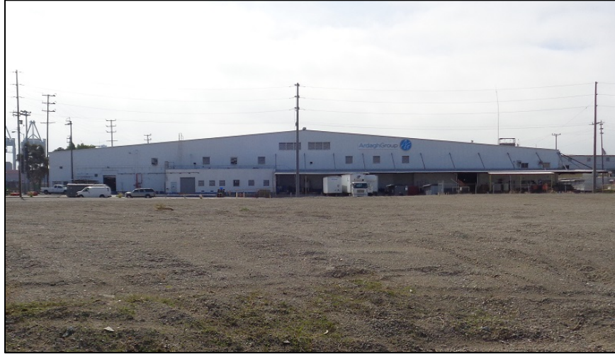
Photograph 1: North elevation, Can Manufacturing (formerly Impress Plant) portion of facility, camera facing south. ICF, 2018.
