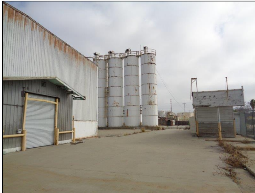
Figure 17: Star-Kist Plant No. 4, south elevation, southeast corner of Plant No. 4 including tanks, camera facing east. ICF, 2018.
