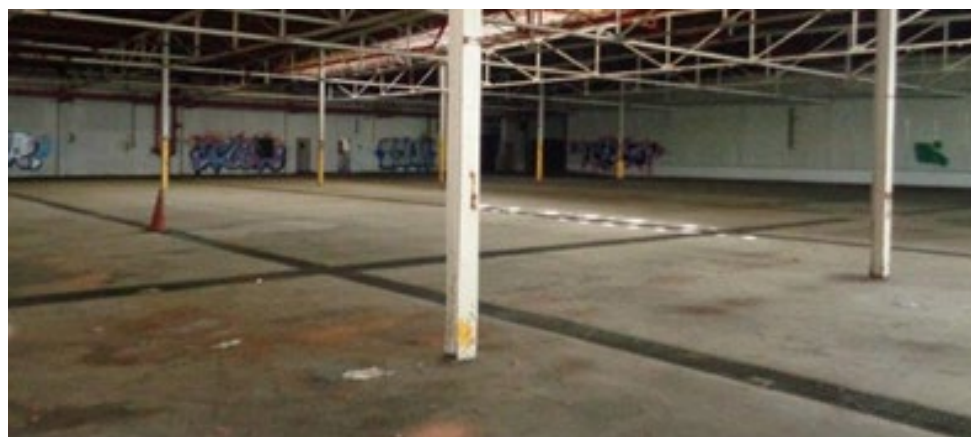
Figure 8-6. Interior in 2018, camera facing southeast.
