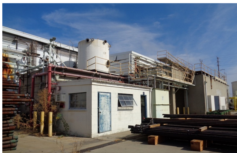
Figure 5-40. South elevation, Cold Storage portion of the facility, camera facing northeast. ICF, 2018.
