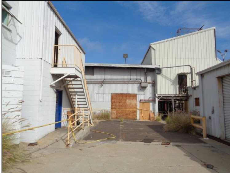
Figure 23: Star-Kist Plant No. 4, rear (east) elevation, detail of ancillary two buildings/structures (left, with staircase; right, with roll-up door) and warehouse/manufacturing building (center), camera facing north. ICF, 2018.
