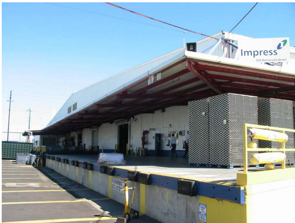
Photo 21. Looking southeast at the northwest corner and northern elevation of the Impress facility
