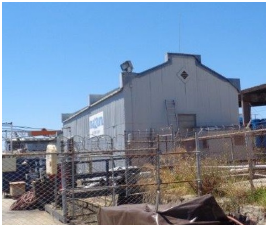
Figure 10-7. 1028 Seaside, Oil Warehouse, east and north elevations, camera facing southwest. ICF, 2020.
