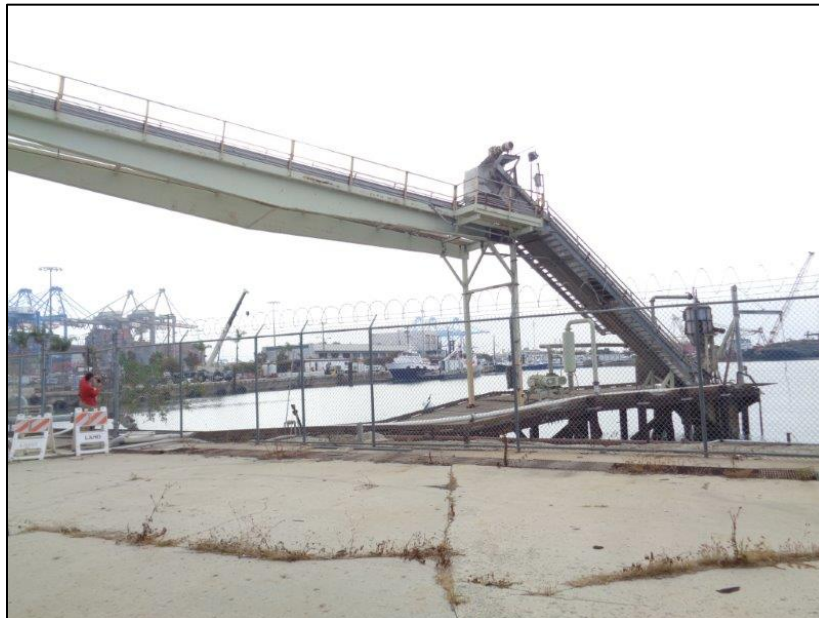
Figure 16: Star-Kist Plant No. 4, ancillary/related buildings/structures adjacent to south elevation, showing the only remaining tuna import bridge and dock, camera facing south. ICF, 2018.
