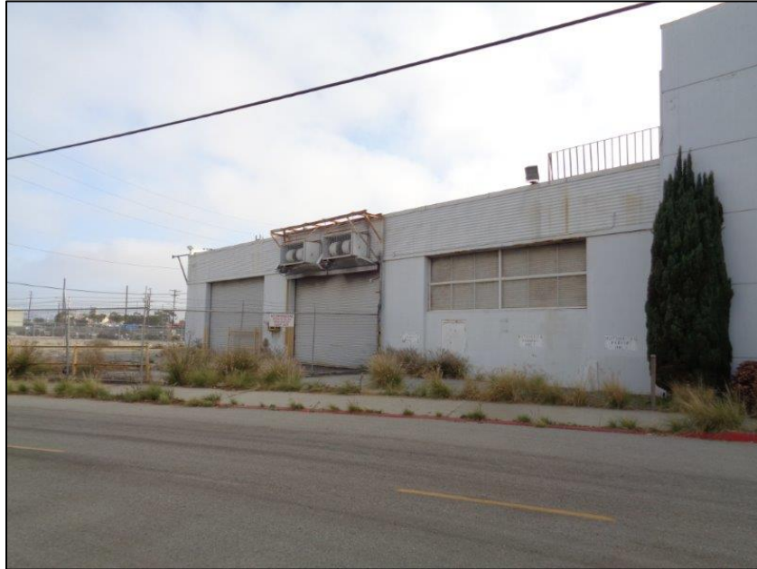
Figure 7: Star-Kist Plant No. 4, primary (west) elevation, detail of northern volume, camera facing northeast. ICF, 2018.
