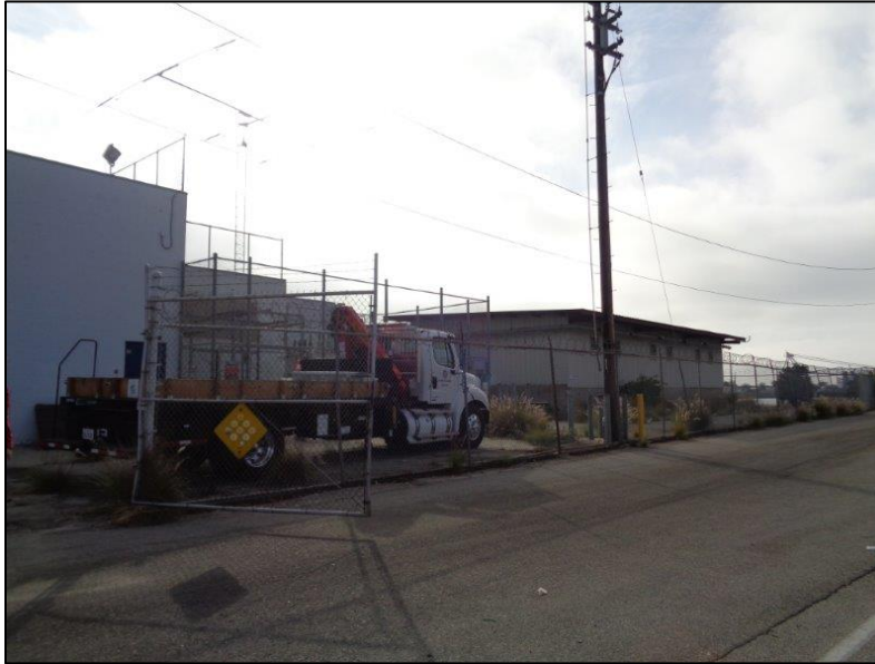
Figure 13: Star-Kist Plant No. 4, primary (west) elevation, detail of southwest corner of Plant No. 4, showing gated electrical area and detached volume, camera facing southeast. ICF, 2018.
