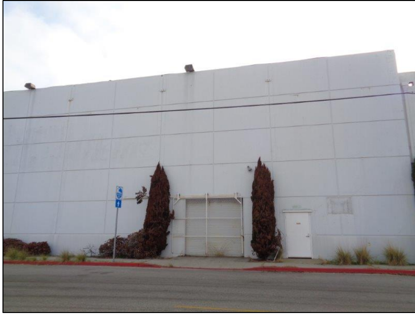
Figure 5-9. Star-Kist Plant No. 4, primary (west) elevation, detail of second volume from the north, camera facing east.
