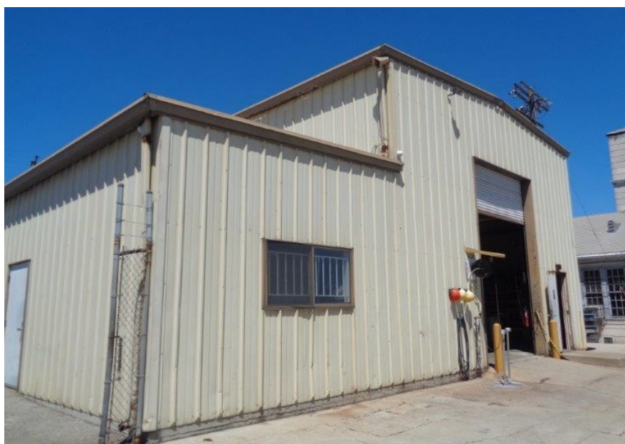
Figure 10-6. East building at 818–980 Seaside Avenue (formerly 906 Seaside Avenue), east and portion of south elevations, camera facing northwest.
