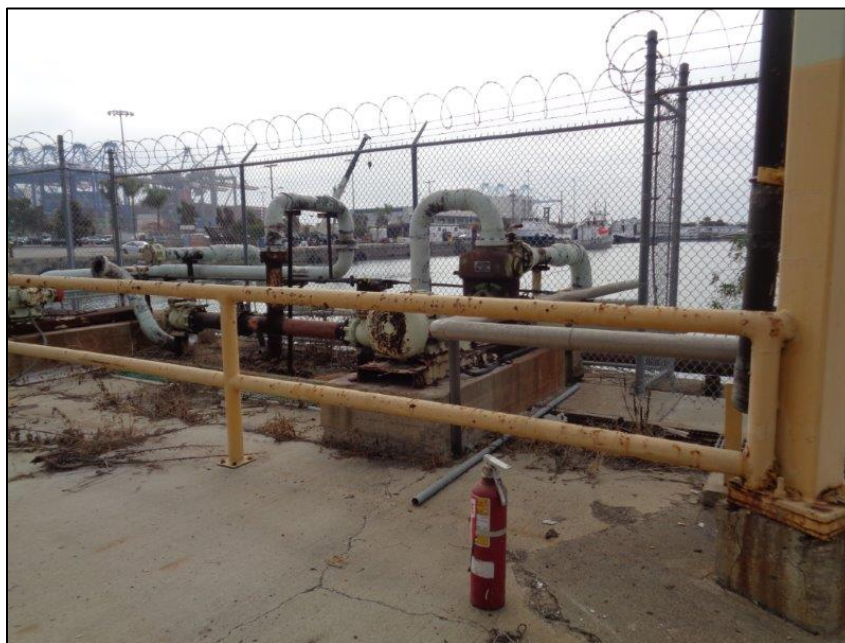
Figure 5-21. Star-Kist Plant No. 4, ancillary/related buildings/structures adjacent to south elevation, showing pipes, railings, fencing, and concrete pads, camera facing southeast.
