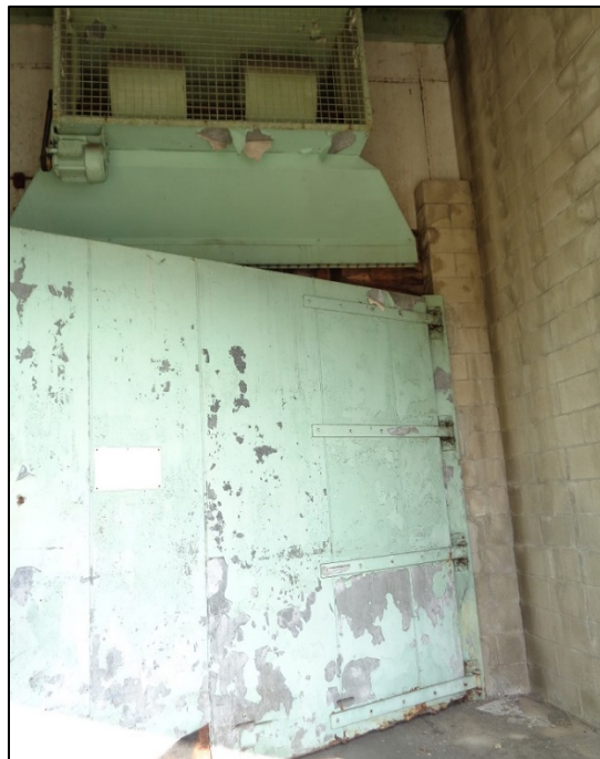
Photograph 6: South elevation, Cold Storage portion of the facility, detail showing a cold storage door, camera facing northeast. ICF, 2018.
