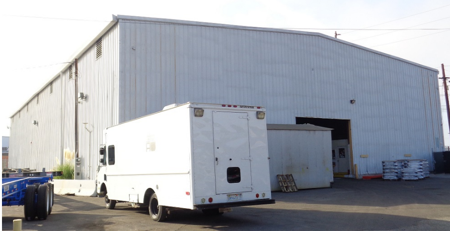
Figure 5-33. North and west elevations, camera facing south.
