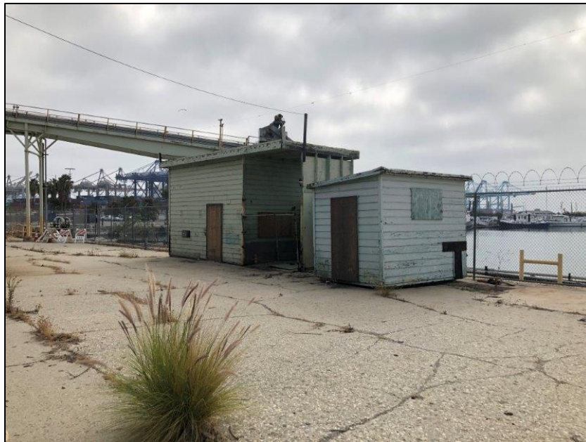
Figure 5-20. Star-Kist Plant No. 4, south elevation's ancillary/related buildings/structures, showing tuna import bridge in background, camera facing southeast.
