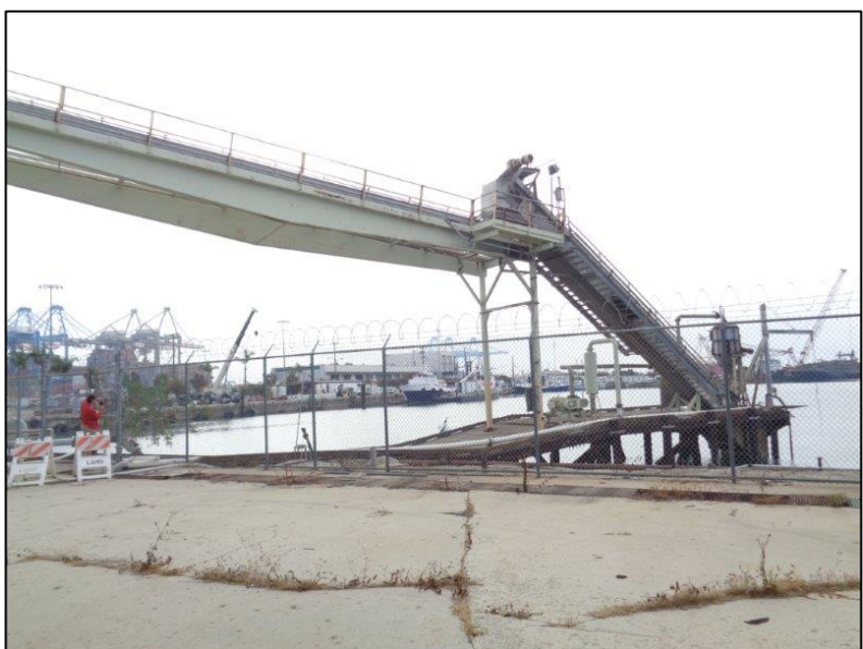
Figure 5-17. Star-Kist Plant No. 4, south elevation’s ancillary/related buildings/structures, showing the only remaining tuna import bridge and dock, camera facing south.
