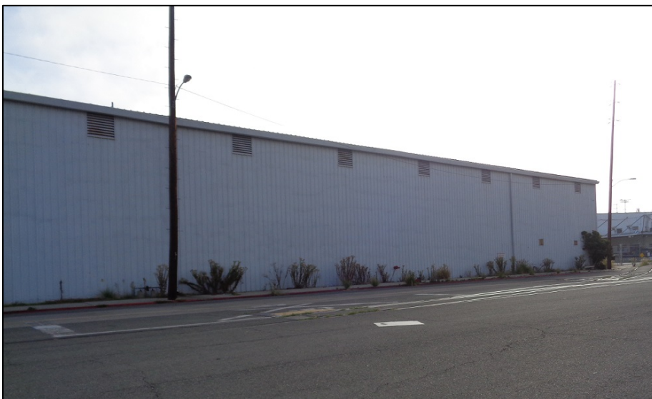
Photograph 2: west elevation, camera facing southwest. ICF, 2018.
