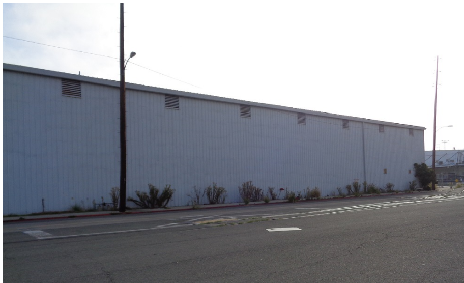
Figure 5-34. West elevation, camera facing southwest.
