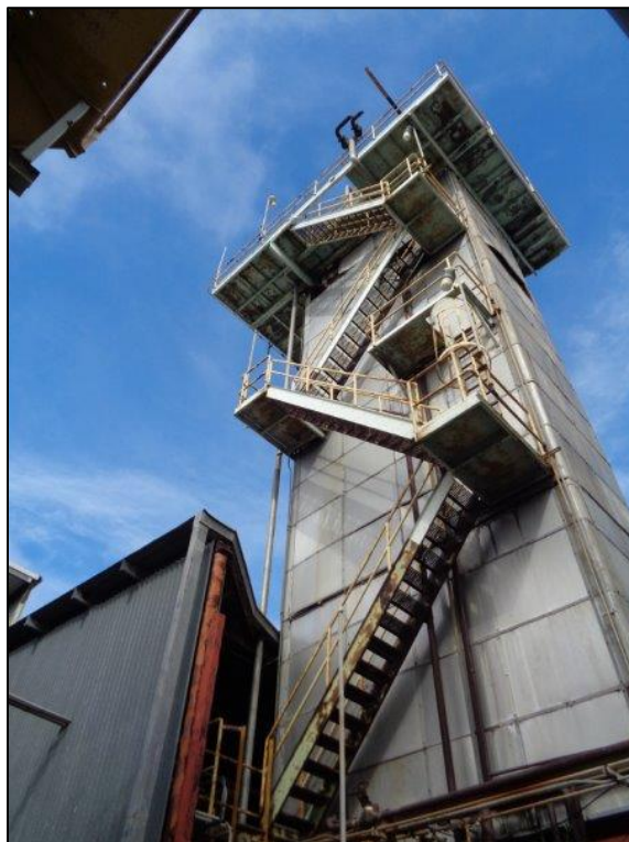
Figure 5-25. Star-Kist Plant No. 4, rear (east) elevation, multi-story tower at center of rear (east) elevation, camera facing north.
