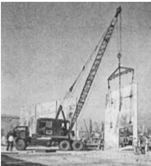
Figure 32: Construction of Star-Kist Plant No. 4. Pan-Pacific Fisherman (December 1952), 18.
