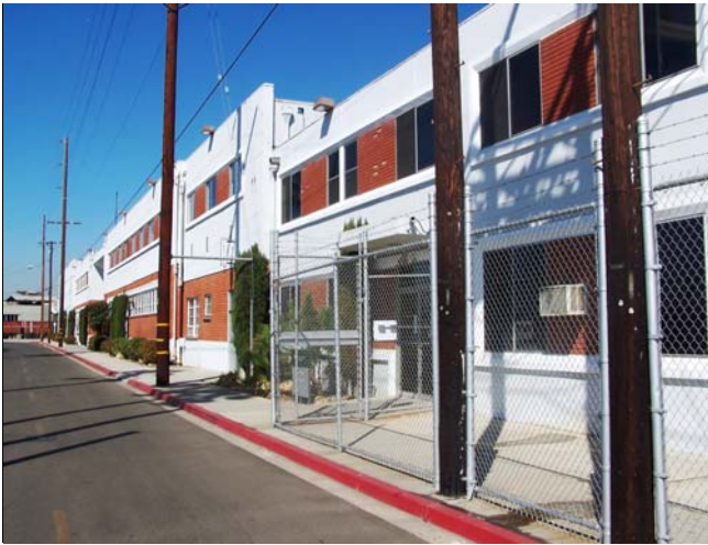
Center of the western elevation of original plant
