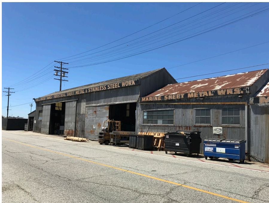
Figure 10-5. DeVries Sheet Metal, primary (west) elevation, camera facing southwest. ICF, 2020.
