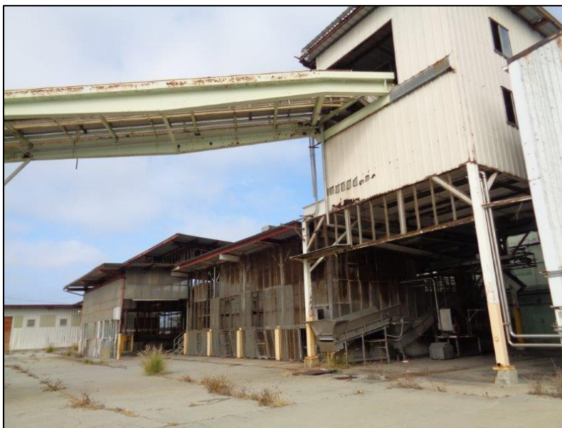
Figure 5-16. Star-Kist Plant No. 4, south elevation, southwest corner of Plant, showing remaining tuna import bridge, camera facing northwest.
