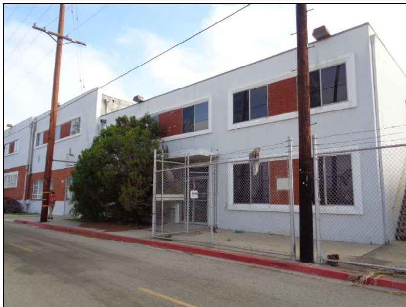
Figure 5-11. Star-Kist Plant No. 4, primary (west) elevation, detail of fifth volume from the north, camera facing northeast.
