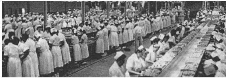
Figure 7-6. Interior, cleaning tables.
