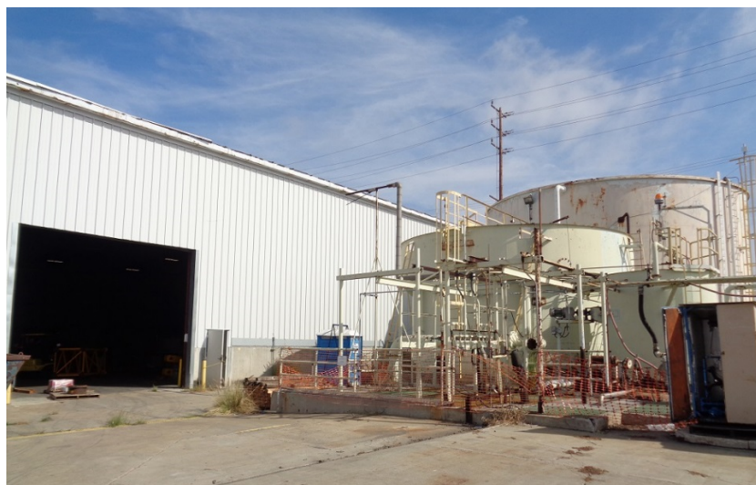
Figure 5-39. South elevation, Cold Storage portion of the facility, camera facing northeast. ICF, 2018.
