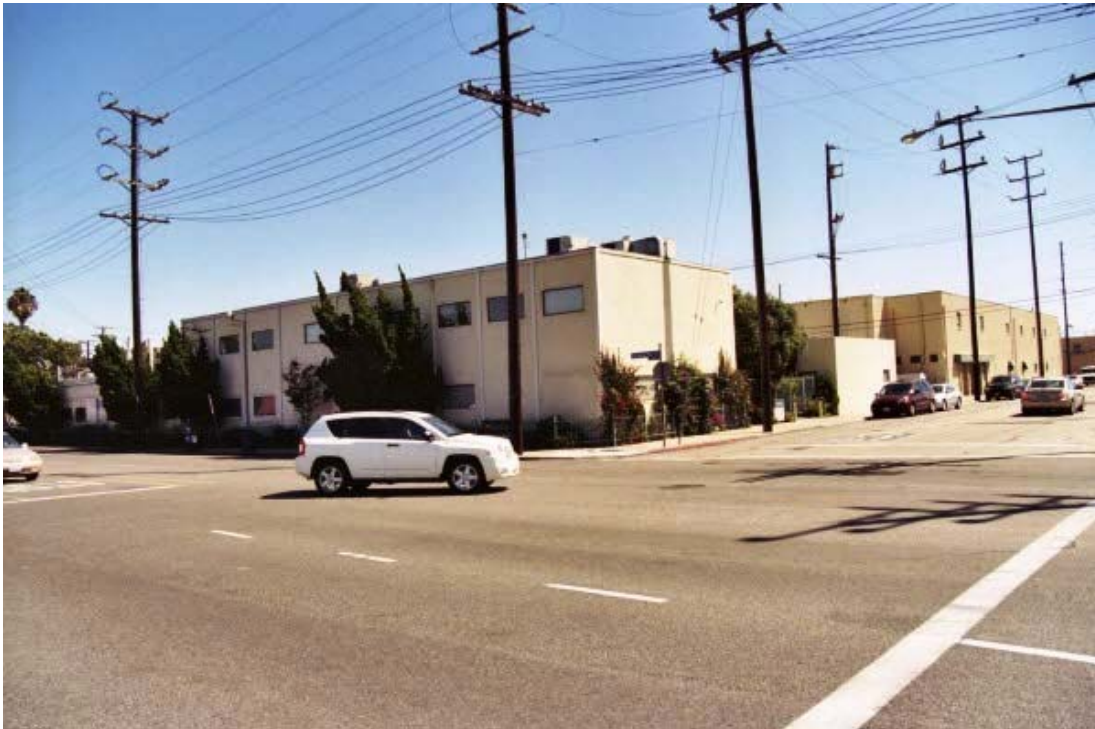
Photo 26. Looking southeast across Terminal Way at the northwestern corner of the Research Laboratory Complex
