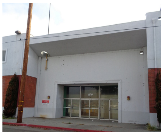
Figure 8-4. Entrance in 2018, camera facing east.
