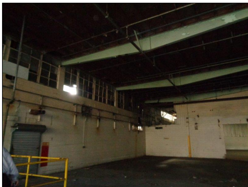
Figure 5-32. Star-Kist Plant No. 4, interior, warehouse/manufacturing area, camera facing southeast. ICF, 2018.
