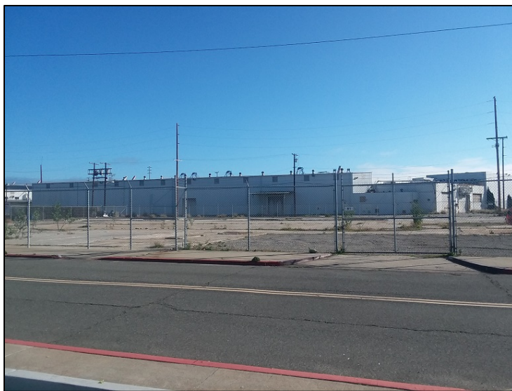
Figure 5-15. Star-Kist Plant No. 4, north elevation, camera facing south. ICF, 2019.
