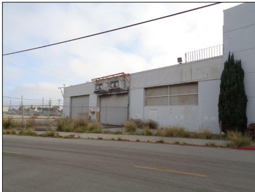
Figure 5-8. Star-Kist Plant No. 4, primary (west) elevation, detail of northern volume, camera facing northeast.
