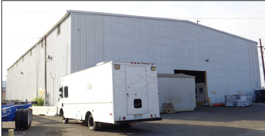
Photograph 1: North and west elevations, camera facing south. ICF, 2018.
