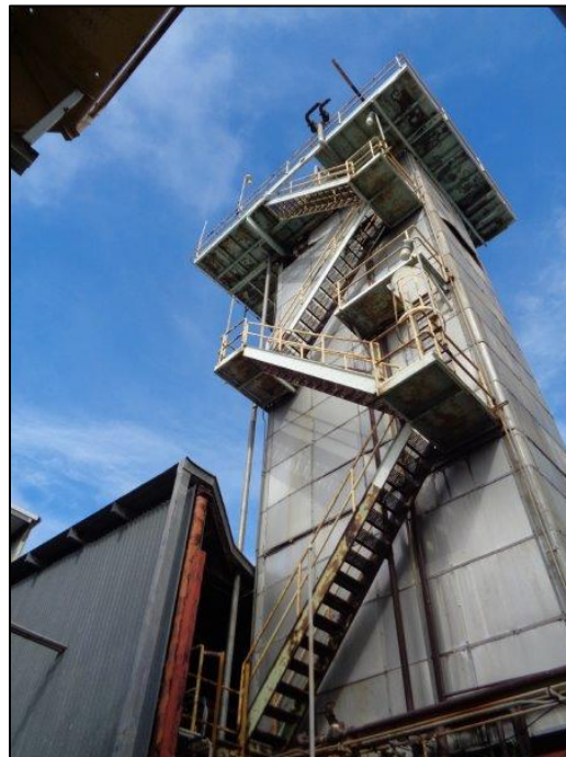
Figure 24: Star-Kist Plant No. 4, rear (east) elevation, multi-story tower at center of rear (east) elevation, camera facing north. ICF, 2018.
