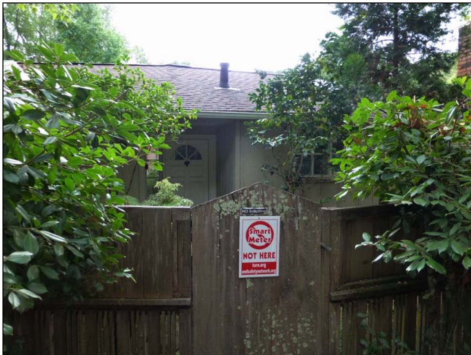
Photograph 3: Detail of entry on west side of residence, facing east, September 20, 2017.
