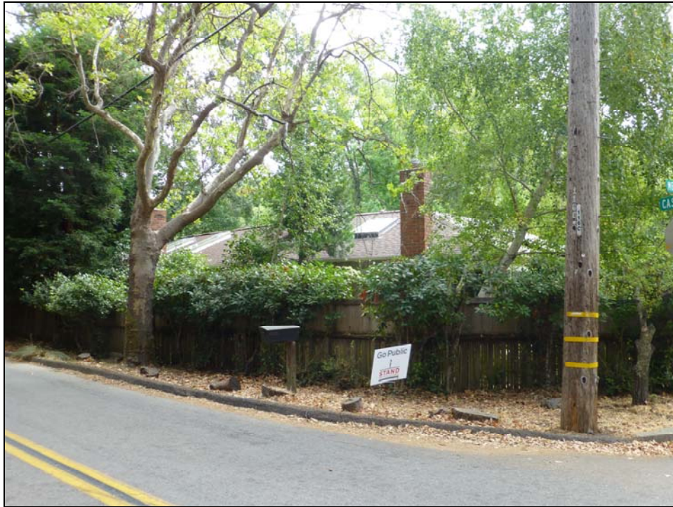
Photograph 2: West side of residence, showing two external chimneys and skylights, facing northeast, September 20, 2017.
