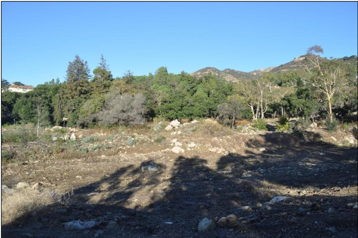
Photo 2. Debris Basin Expansion Area from East Mountain Drive, Looking Northwest
