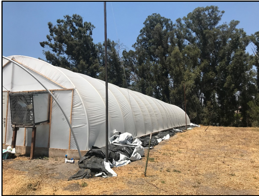
Photo 1. Existing hoop house structure adjacent to Drainage 1, view north (August 6, 2018).
