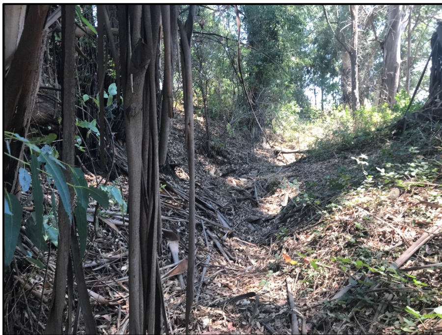
Photo 2. Drainage 1 along the northern boundary of the project site, view east (August 6, 2018).
