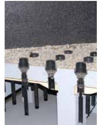
6 Filtration Anthracite Coal Filters, LAAF Water passes through 60 inches of anthracite coal filters, which remove particles smaller than can be seen through a microscope.
