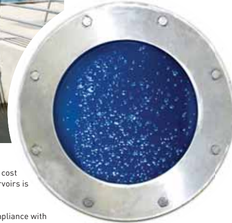
6 Filtration Anthracite Coal Filters, LAAF Water passes through 60 inches of anthracite coal filters, which remove particles smaller than can be seen through a microscope.
