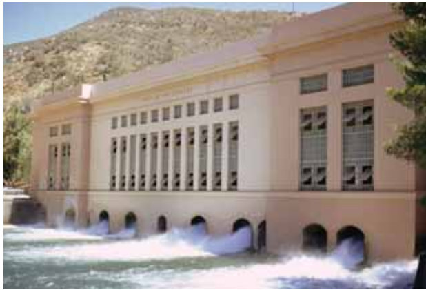
2 Making Hydropower San Francisquito Power Plant 1 Water generates electricity as it passes through the hydroelectric plant
