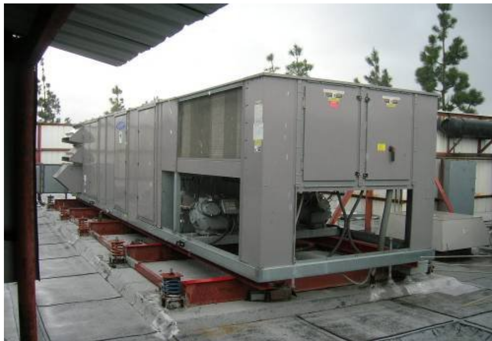
View of one of two large air conditioning systems installed on the roof of Bldg F6 at the Subject. Bldg F5 HVAC systems are identical to this.
