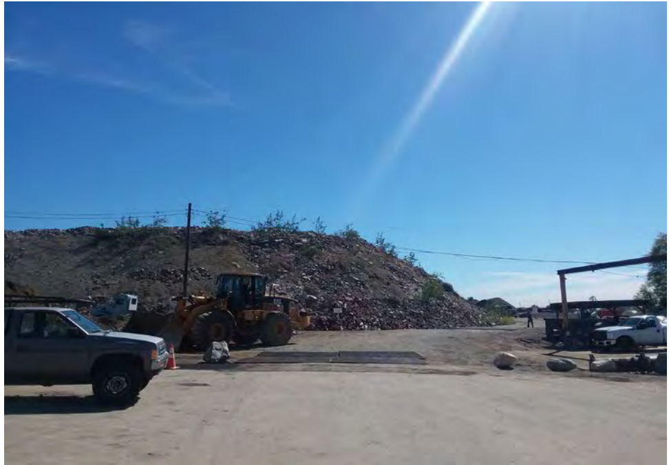
Photograph No. 1: Entrance to the site from Airport Drive, looking east.
