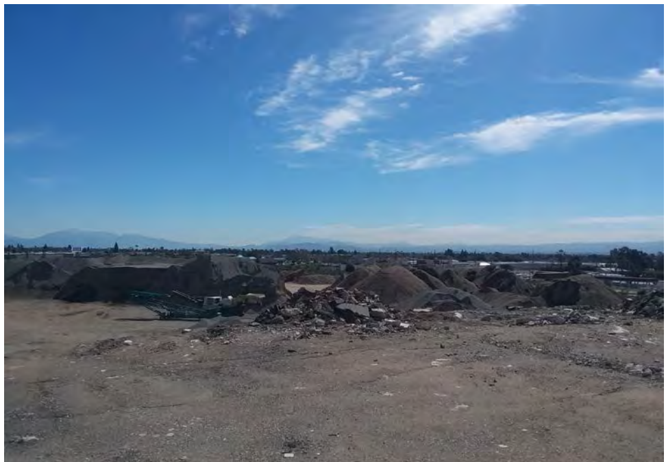
Photograph No. 2: Typical sand and rock stockpiles segregated by grain size.
