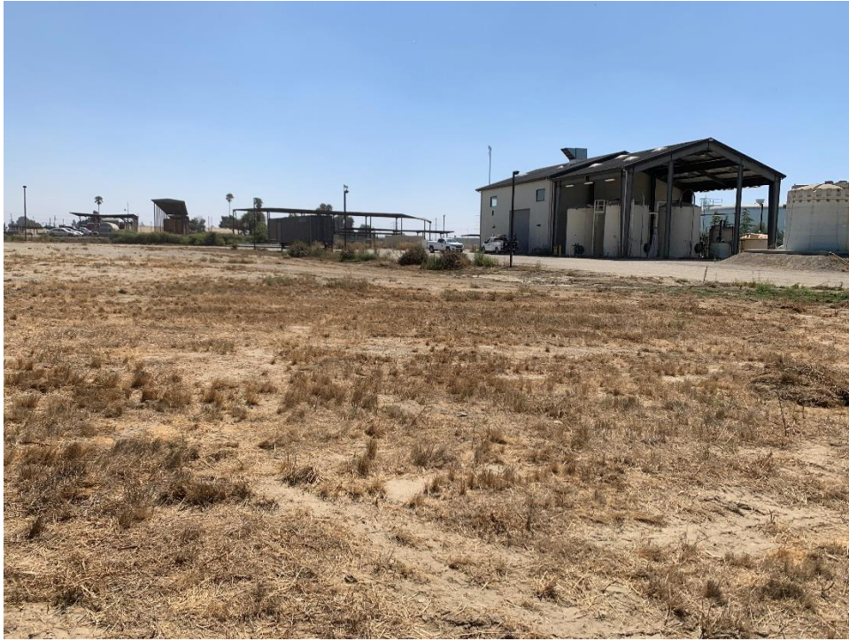
Figure 5-1 Overview of existing facility on Schaefer Avenue, view to the east
