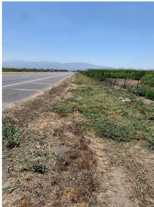
Figure 5-4 Preferred Alignment along Euclid Avenue, view to the south
