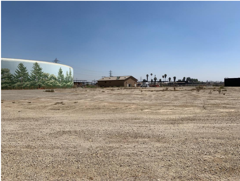
Figure 5-2 Overview of existing facility on Schaefer Avenue, view to the southwest
