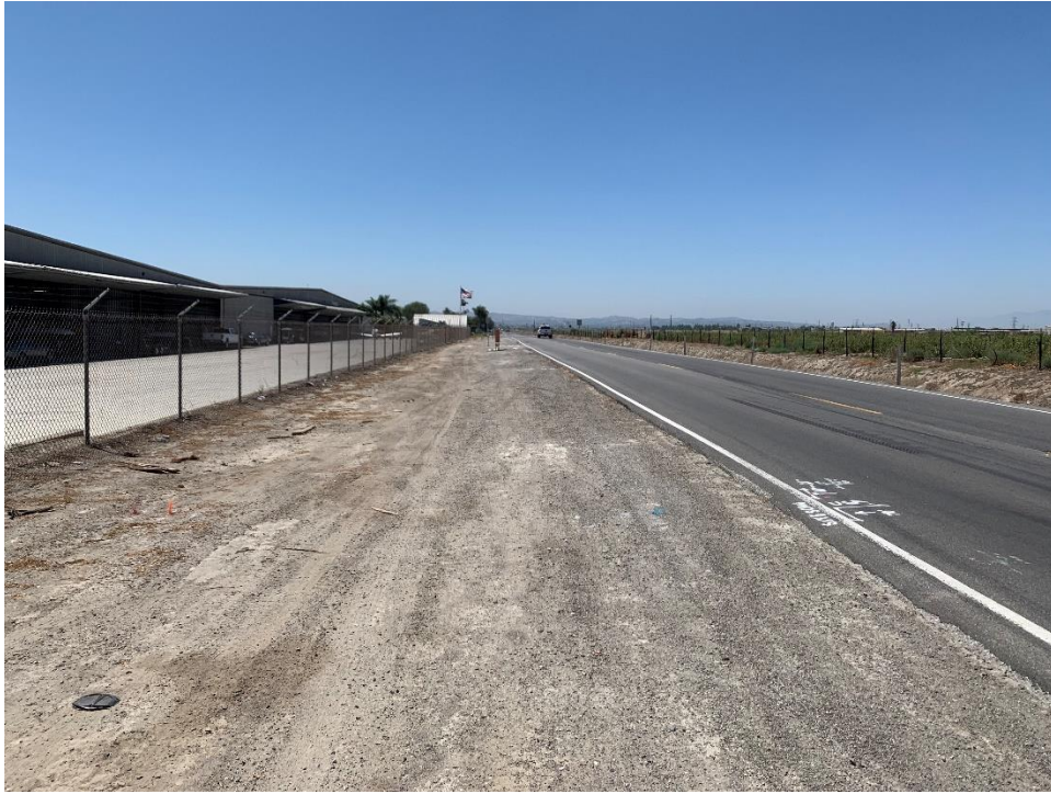
Figure 5-5 Preferred Alignment along Merrill Avenue, view to the north
