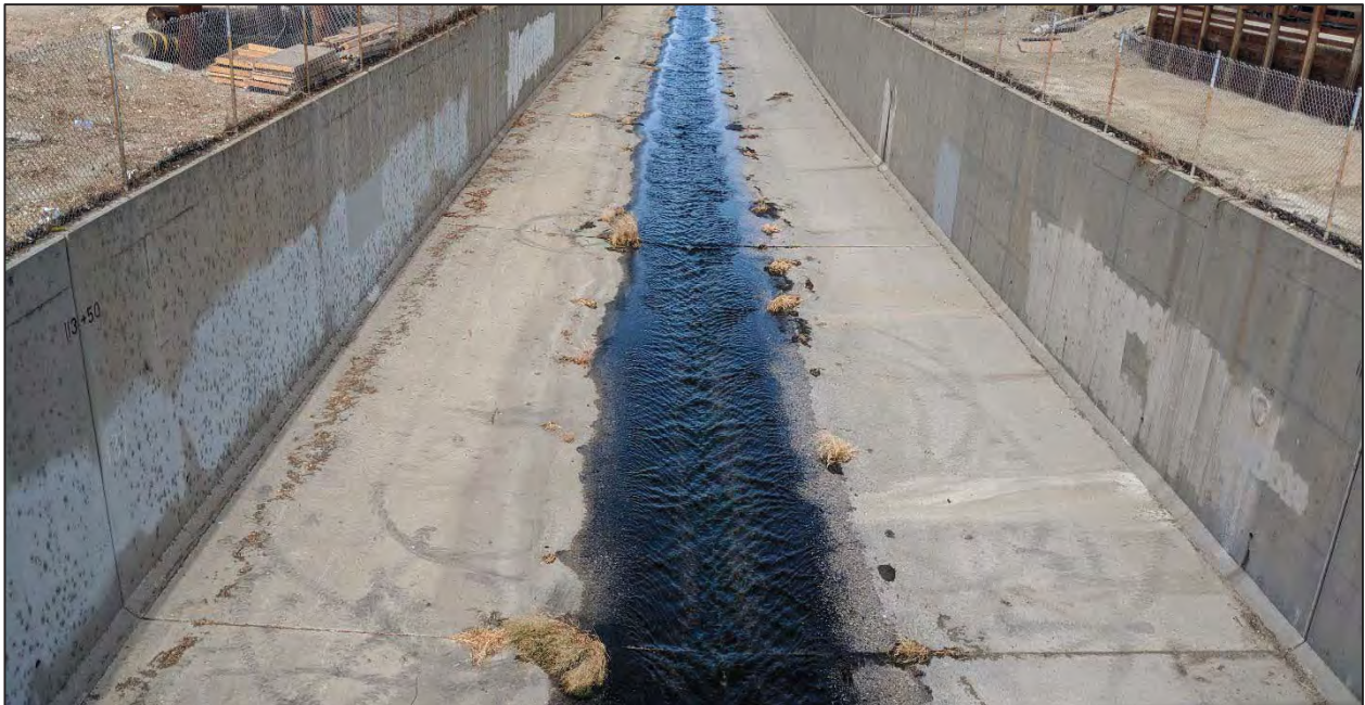
Photograph 2: Representative photograph showing the Burbank Western Channel
