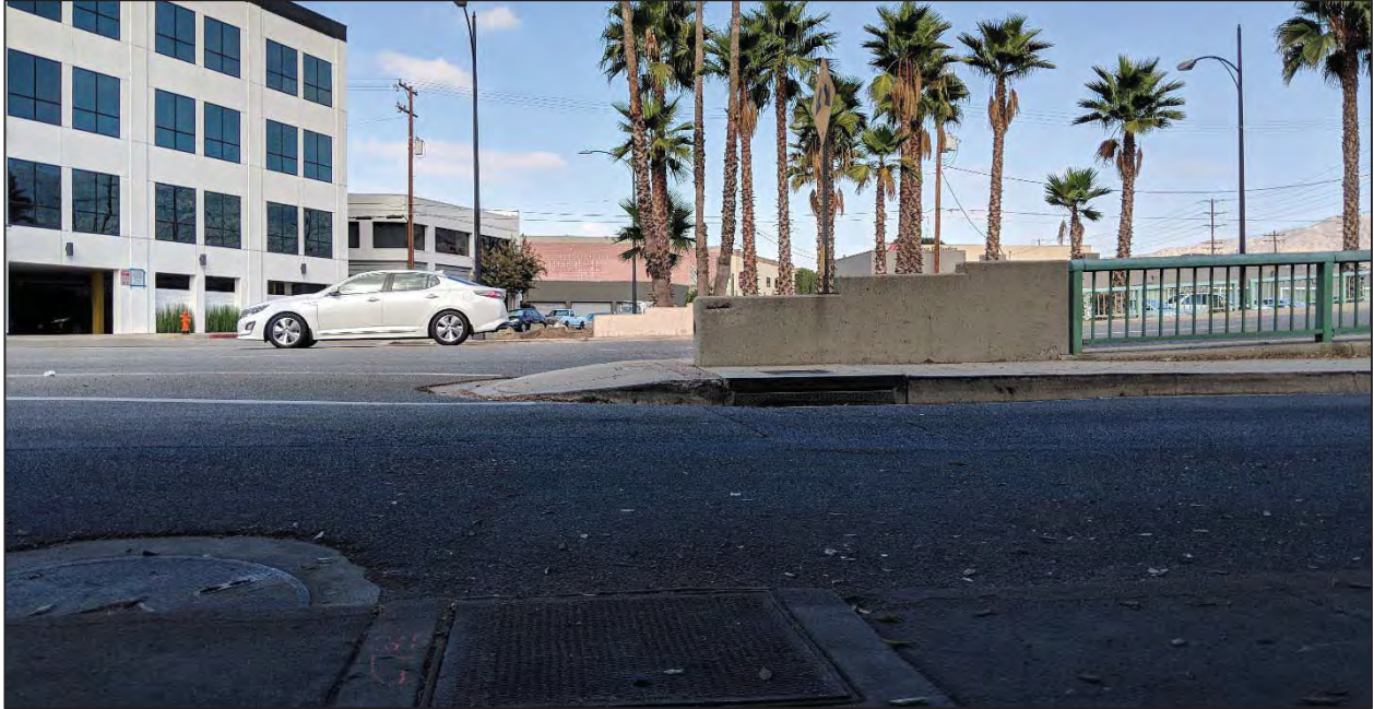
Photograph 1: Representative photograph showing location of current stormwater system currently connecting adjacent property to Project Site
