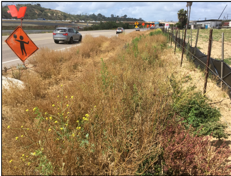
PHOTOGRAPH 1 Looking Southwest at Drainage Ditch Adjacent to Manchester Avenue
