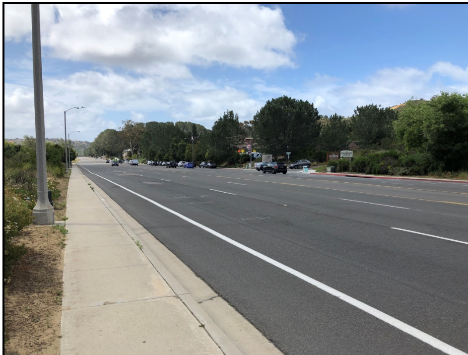
PHOTOGRAPH 4 Looking South on El Camino Real North of the Manchester Avenue/El Camino Real Intersection
