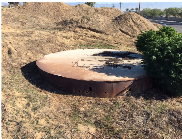
Photo 1: Steel Tank. View Northeast.
