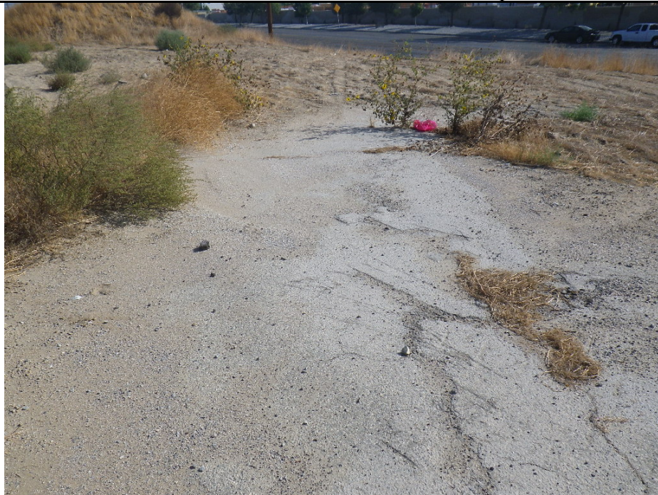
Photo No. 19 – Northeast view of pavement in site's southeastern portion.
