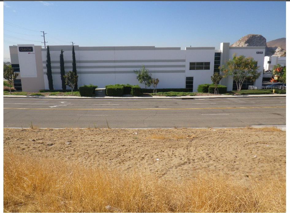
Photo No. 26 – South view of commercial/lt. industrial building south of site.
