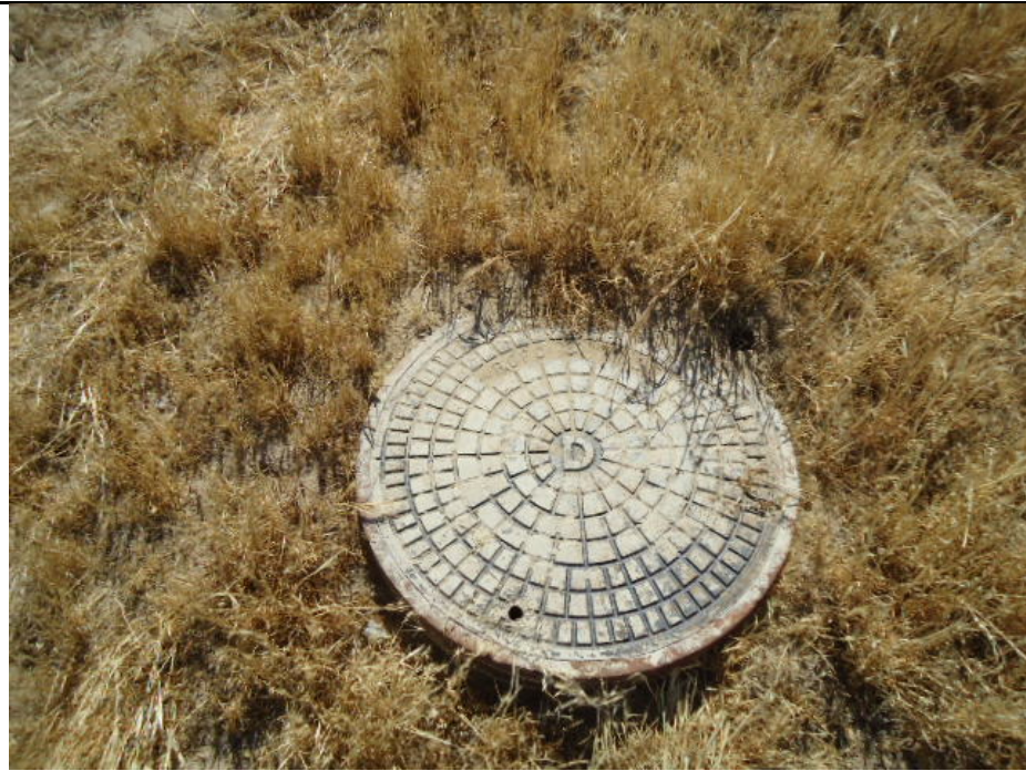
Photo No. 5 – View of manhole cover in site's northwestern portion.
