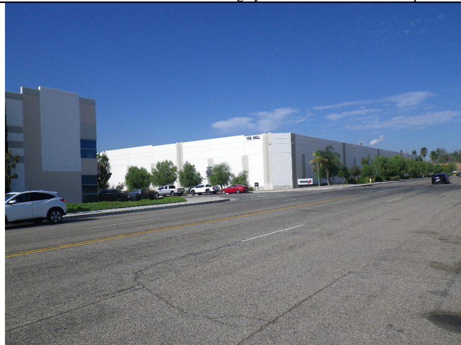
Photo No. 27 – SW view of commercial/lt. industrial buildings south of site.
