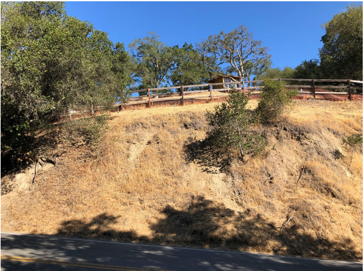
Same roadcut as above, adjacent to north (right) side of large Oak tree. Note sporadic nature of exposures of nearly vertical Ladera Formation subunits (see Figure 5) (Photo credit: CSH, 2021)
