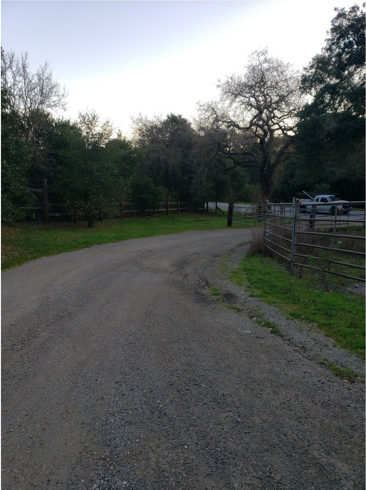
Figure B-1. Photo 1, gated entry into Project site, facing northeast towards Alpine Road.
